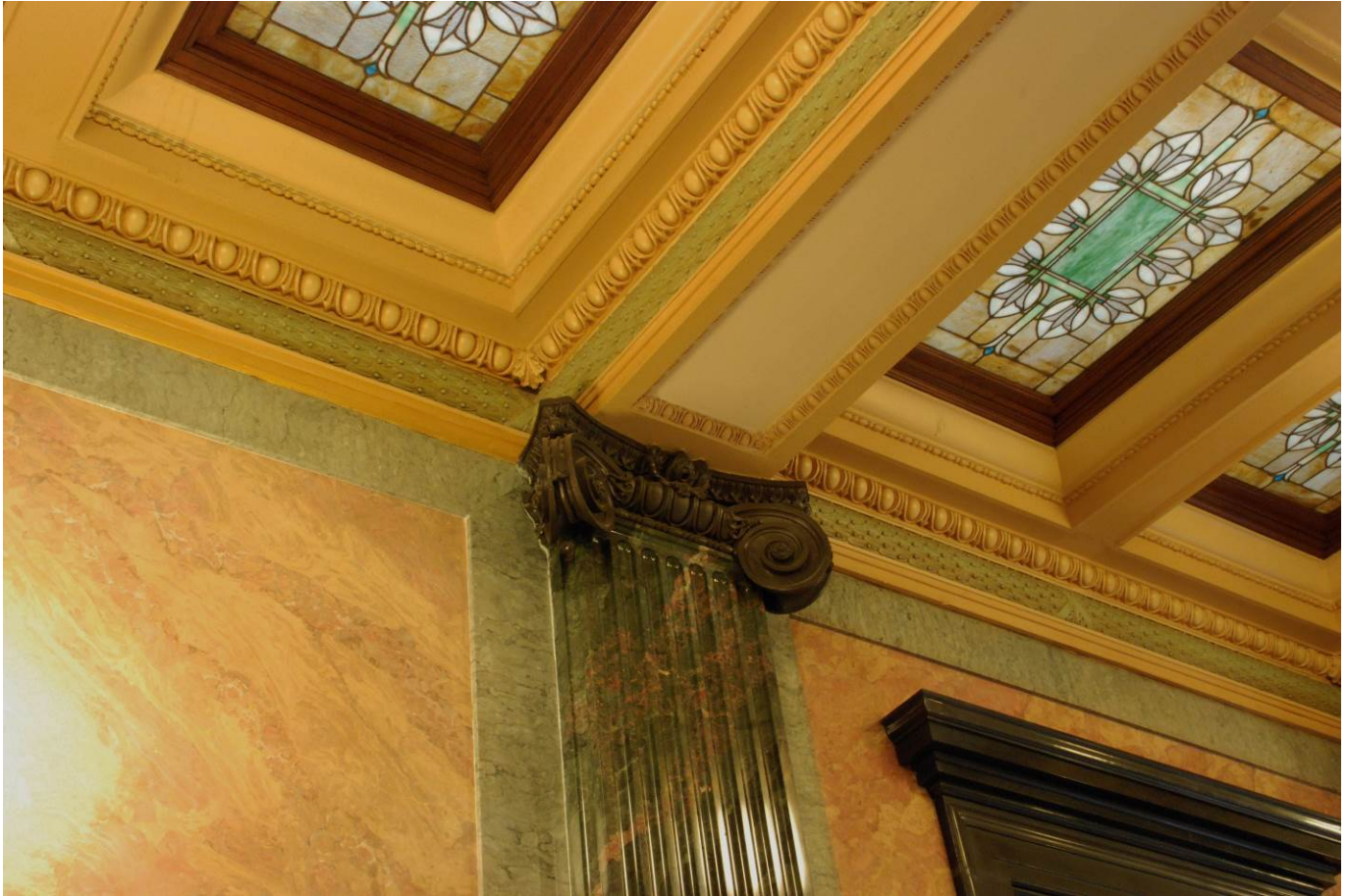
Fig. 12. Mississippi State Capitol. Detail of the wall and ceiling of the third-floor corridor, showing the scagliola wall surfaces, an Ionic pilaster, and three of the art glass panels in the ceiling that transmit light from the story above. Jennifer Baughn, photographer, 2012 (Mississippi Department of Archives and History).
