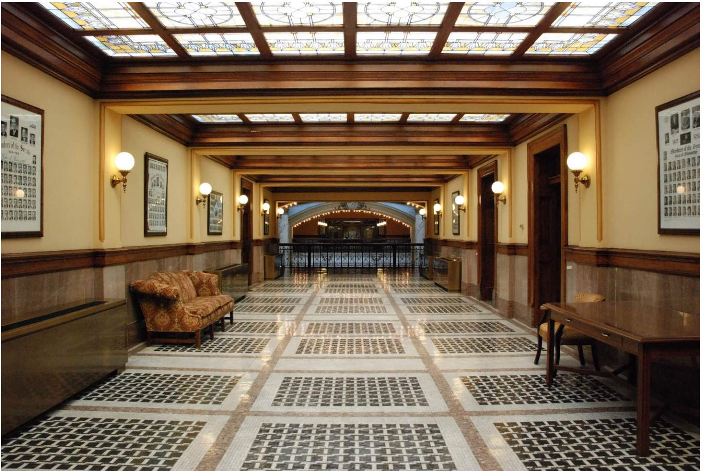
Fig. 18. Mississippi State Capitol. The fourth-floor eastern corridor, showing the glass blocks set into the floor to transmit light from the skylights to the story below. Jennifer Baughn, photographer, 2012 (Mississippi Department of Archives and History).
