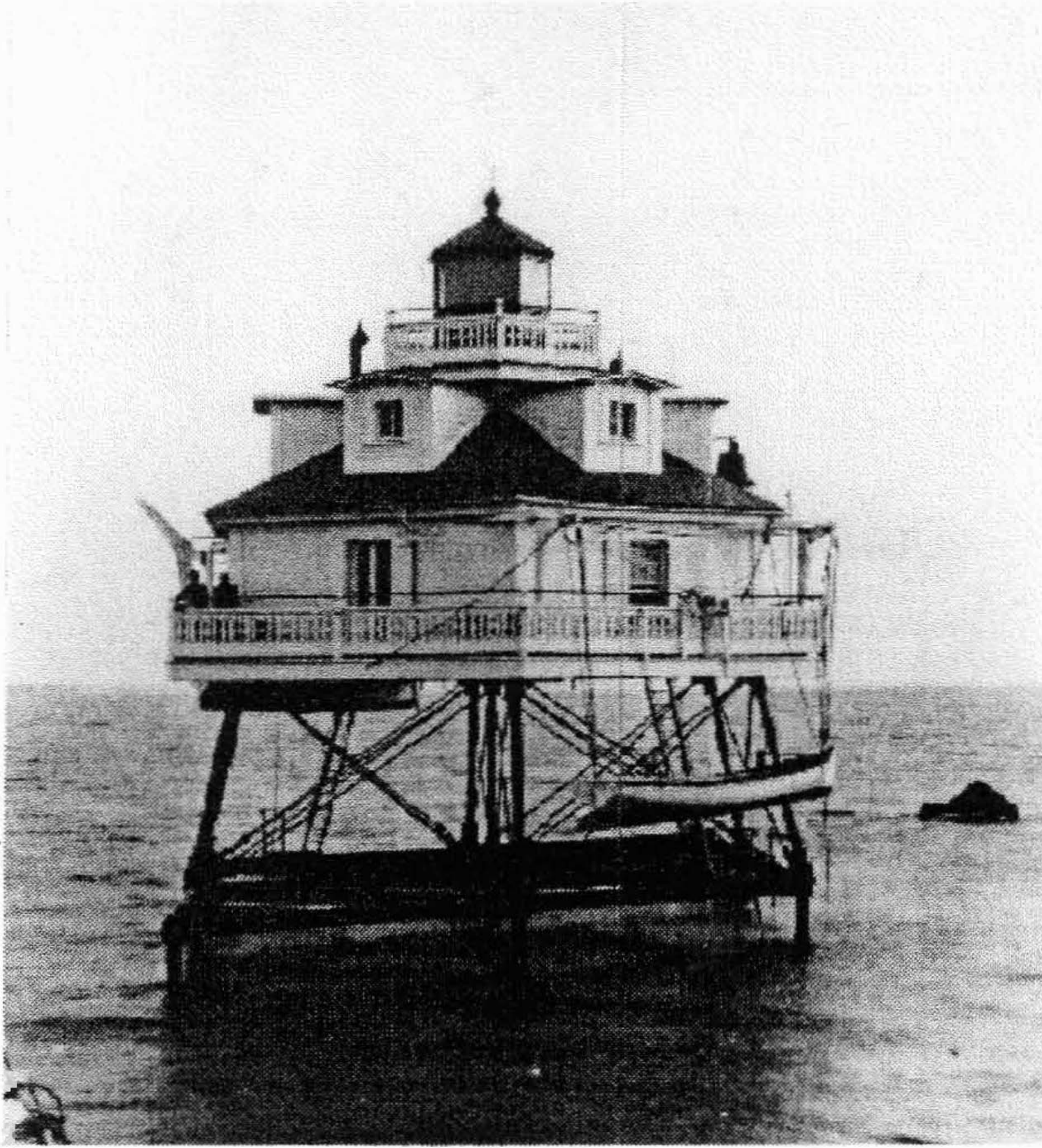
Thomas Point Shoals Lighthouse with screwpile foundation located in Maryland's Chesapeake Bay; shown here in 1885.
