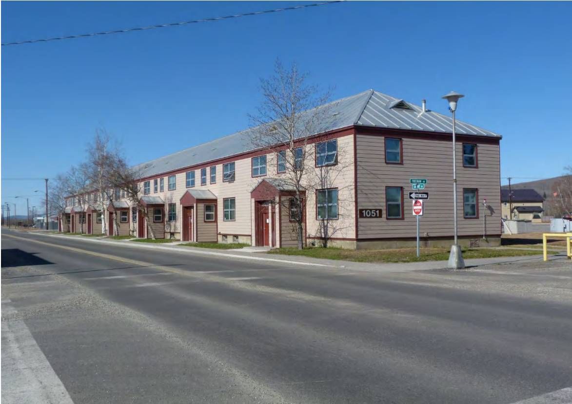
Photo 10 of 18. Building 1051 (Officers' Quarters), 2016, view to the northwest.
