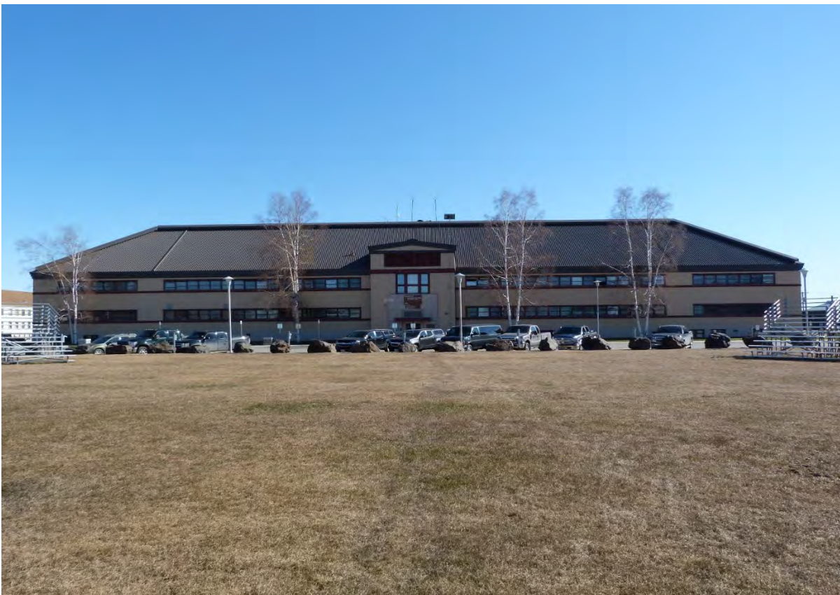
Photo 13 of 18. Building 1555 (Barracks and Post Hospital), 2016, view to the east.
