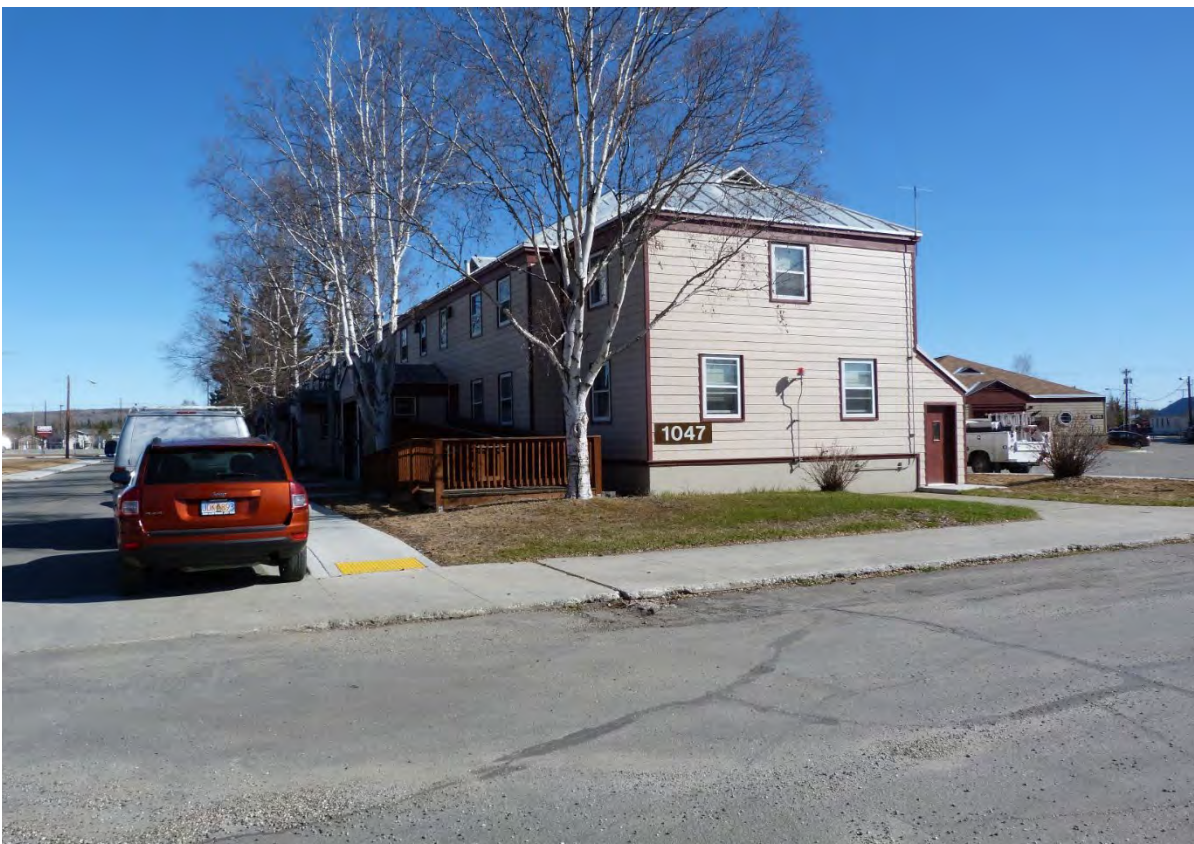
Photo 7 of 18. Building 1047 (Officers' Quarters), 2016, view to the west.
