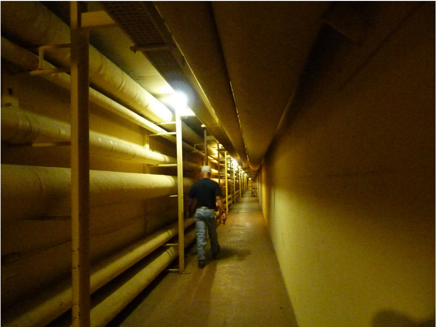
Photo 18 of 18. Utilidor, interior passageway, 2017.
