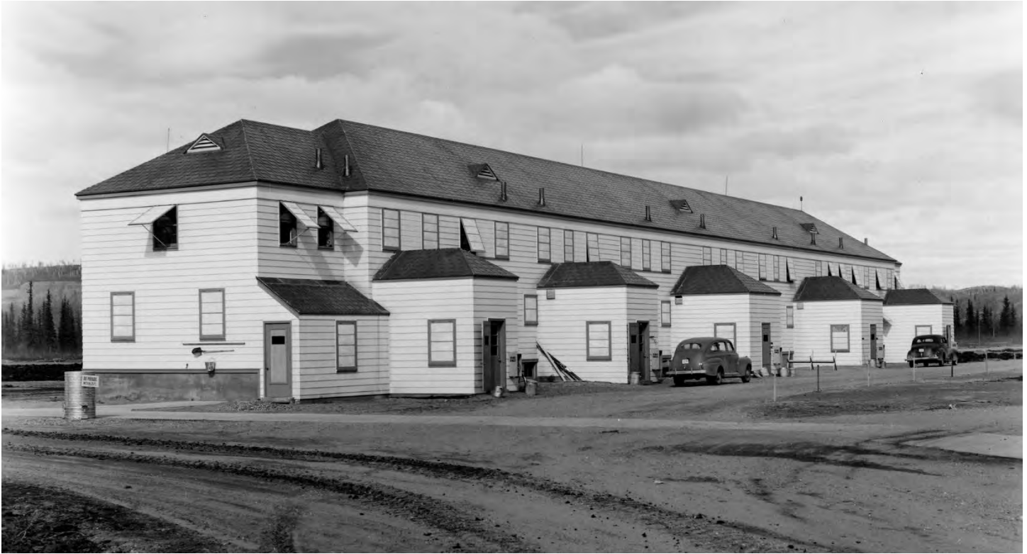
Figure 5. Officers' Quarters (Building 1047), 1942.
