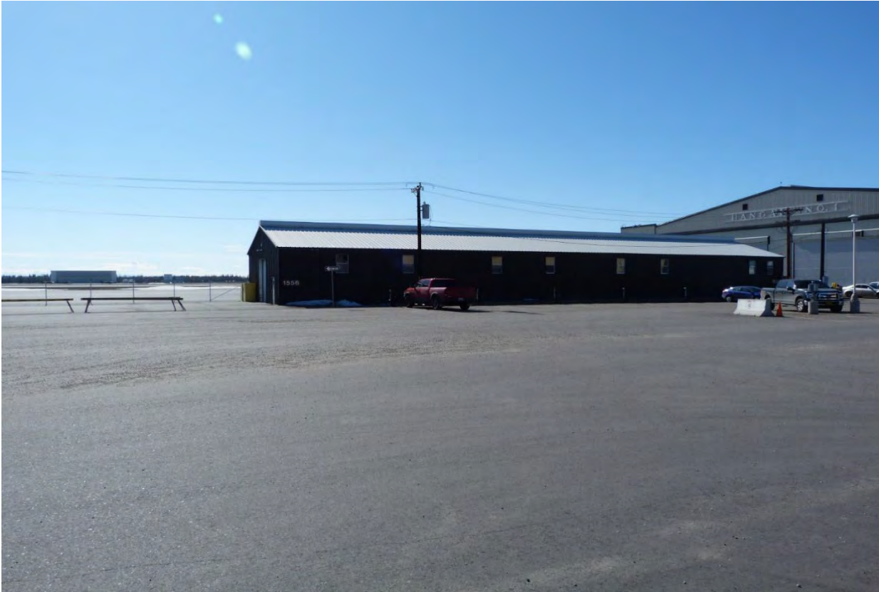
Photo 14 of 18. Building 1556 (Butler Building), 2016, view to the south.
