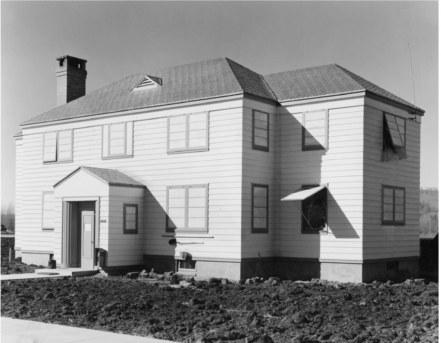
Figure 6. Commander's Quarters (Building 1048), 1942.
