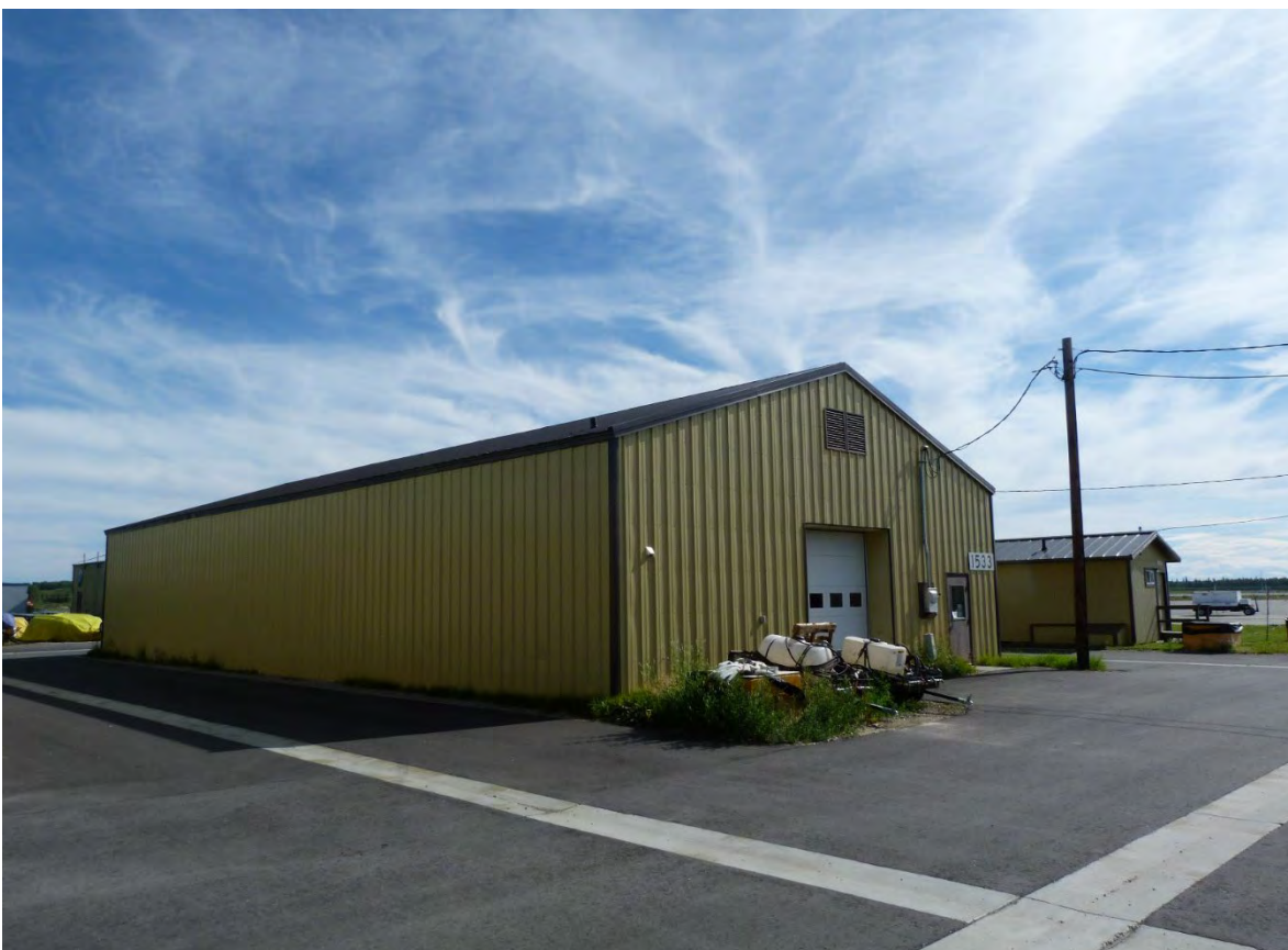
Photo 11 of 18. Building 1533 (Butler Building), 2016, view to the southeast.
