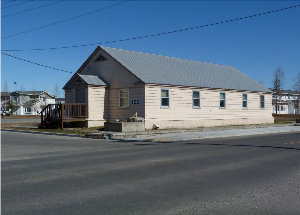
Photo 2 of 18. Building 1021 (Nurses' Quarters), 2016, view to the northeast.
