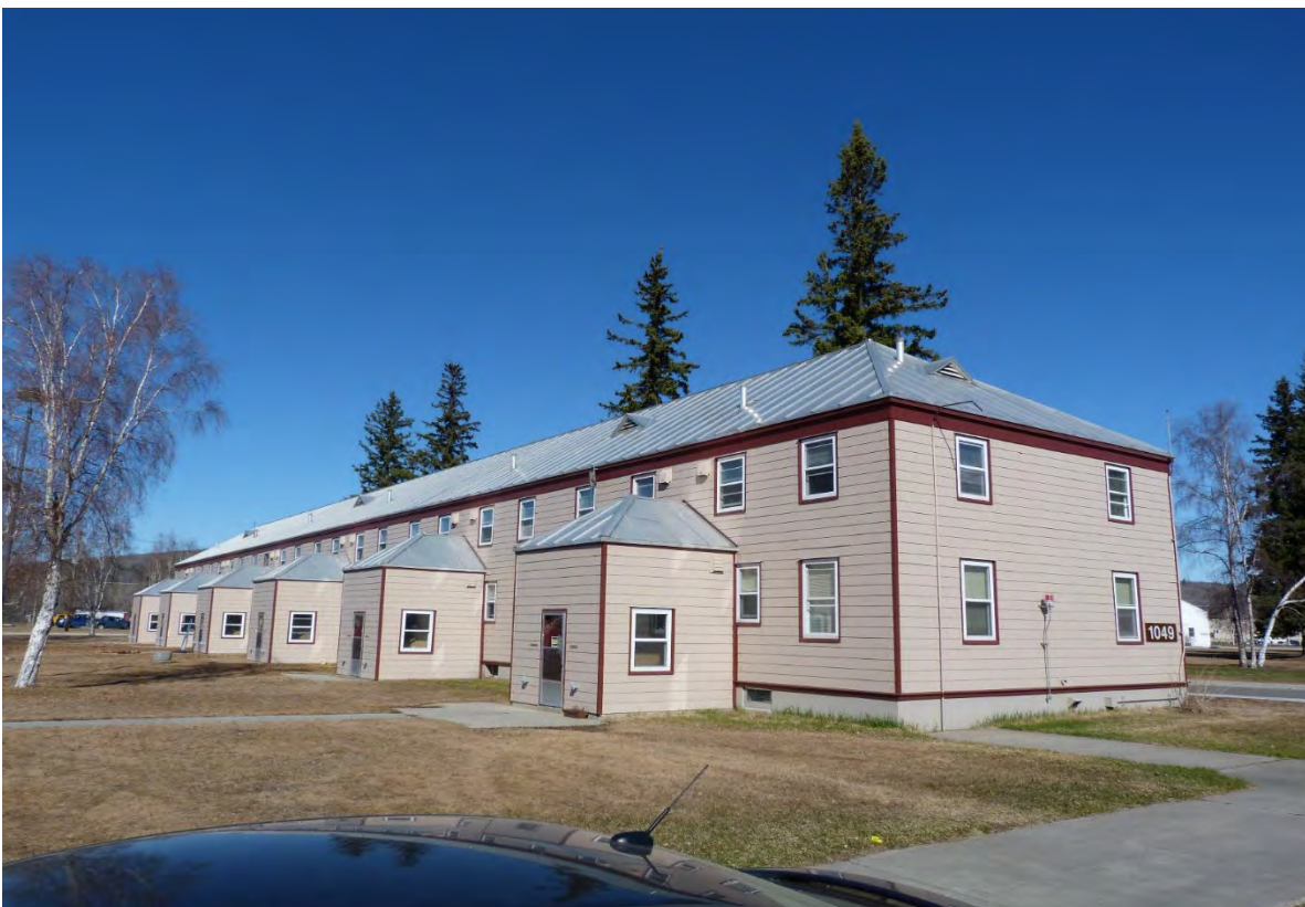
Photo 9 of 18. Building 1049 (Officers' Quarters), 2016, view to the west.
