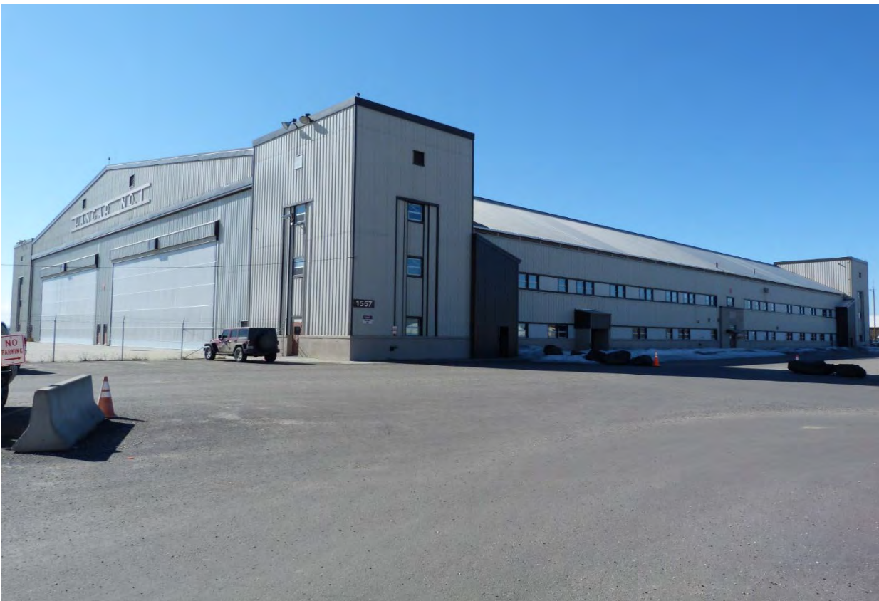
Photo 15 of 18. Building 1557 (Hangar 1), 2016, view to the southwest.
