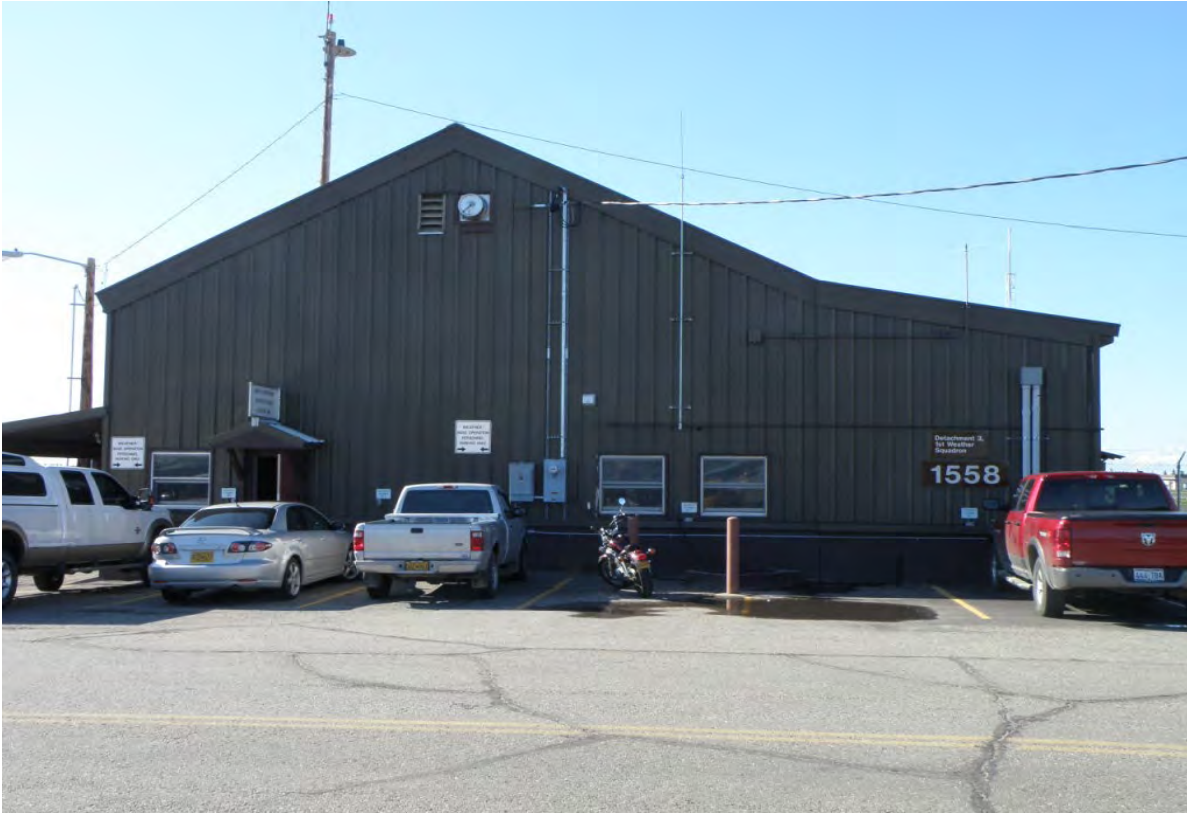
Photo 16 of 18. Building 1558 (Butler Building), 2016, view to the south.
