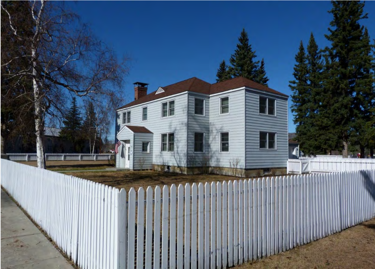
Photo 8 of 18. Building 1048 (Commander's Quarters), 2016, view to the northwest.
