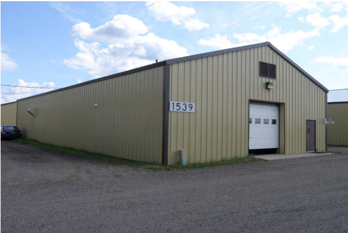
Photo 12 of 18. Building 1539 (Butler Building), 2016, view to the northwest.
