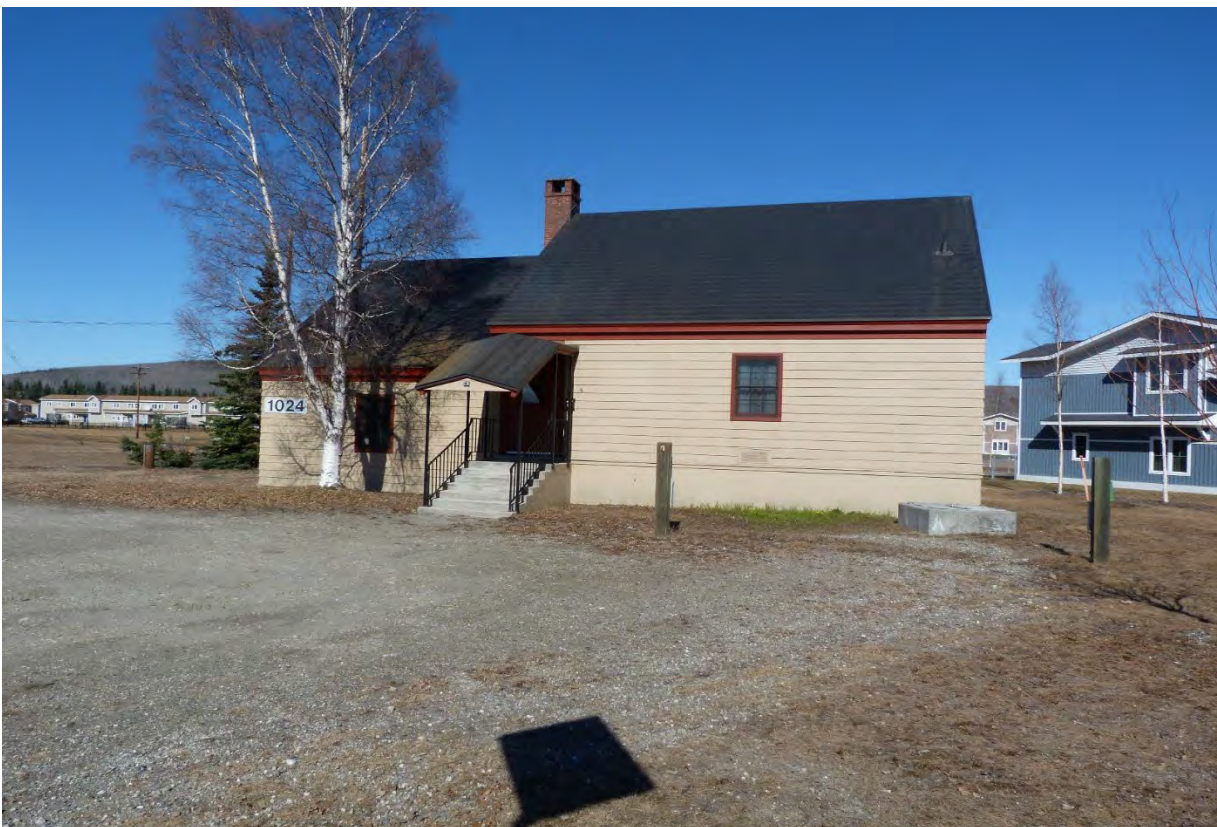
Photo 3 of 18. Building 1024 (MARS Building), 2016, view to the north.
