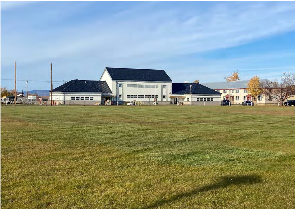
Photo 17 of 18. Building 1562 (Quartermaster Warehouse), 2022, view to the southwest.
