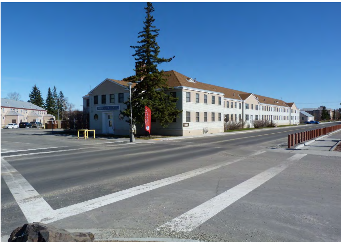
Photo 5 of 18. Building 1045 (Murphy Hall), 2016, view to the northeast.
