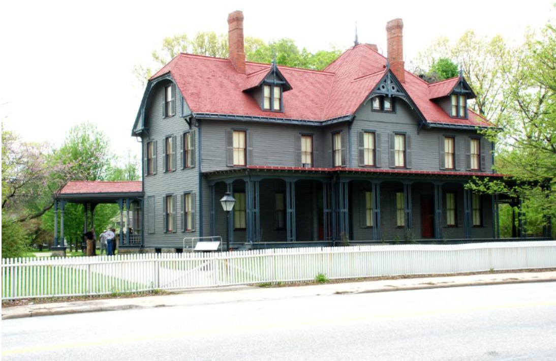
James A. Garfield Home, Main House, Main (South) Elevation Photo by Robert W. Blythe, May and December 2014
