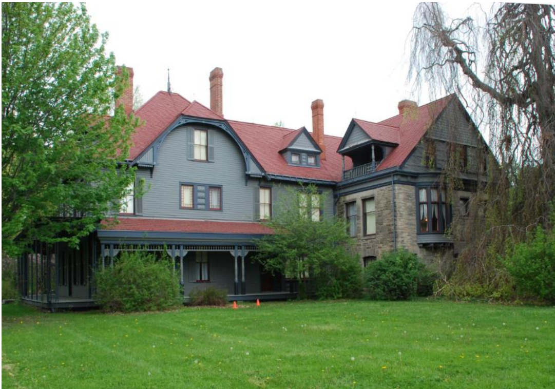
James A. Garfield Home, Main House, East Elevation Photo by Robert W. Blythe, May and December 2014
