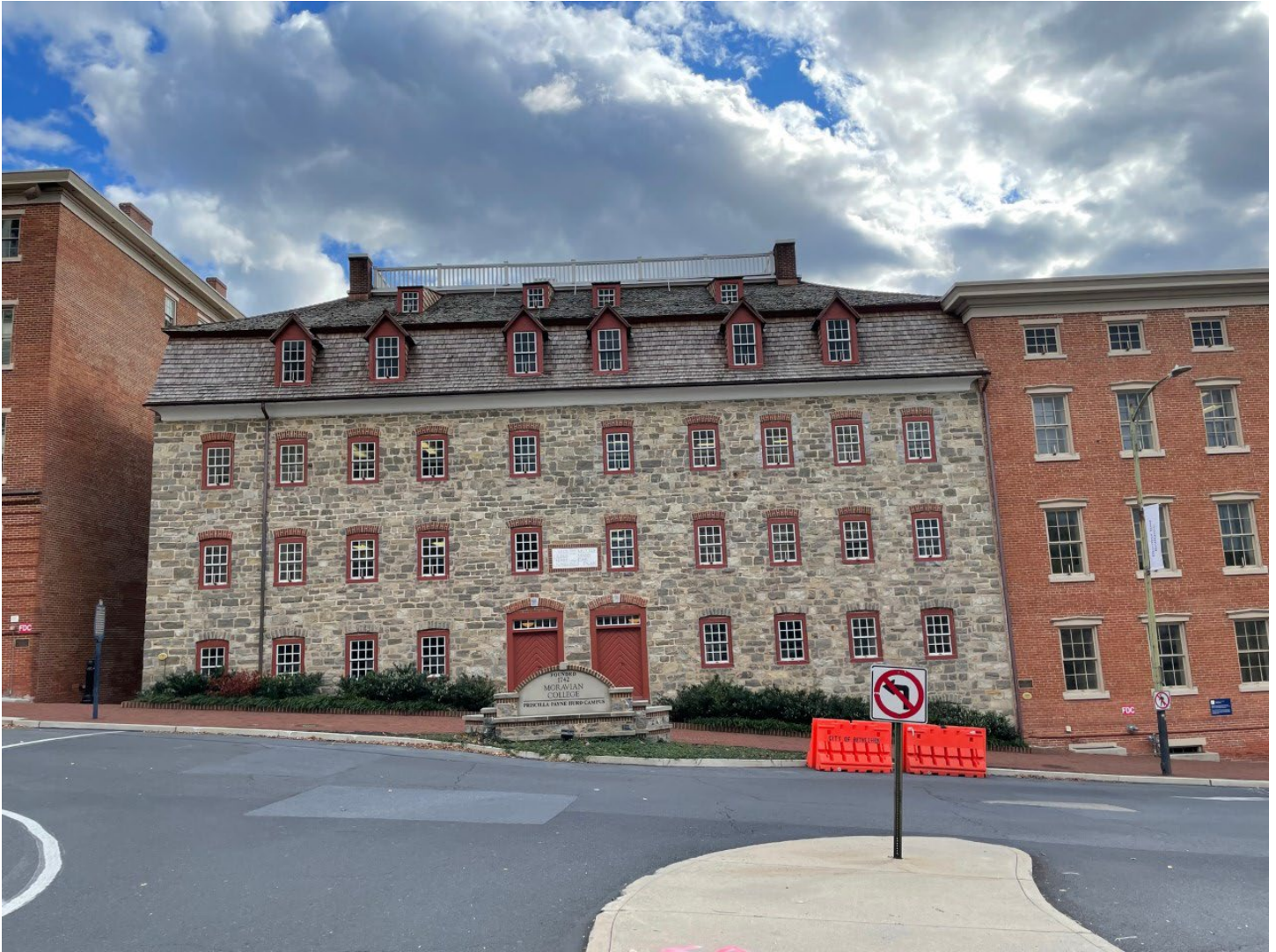
1748 Single Brethren's House Historic Moravian Bethlehem Historic District Front elevation looking South Photo by Catherine Turton, NPS, 2021
