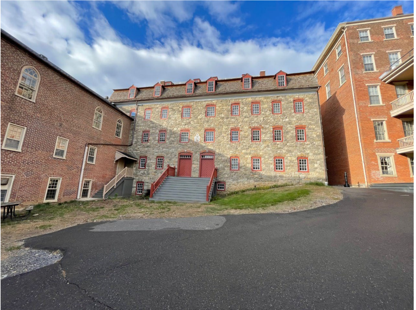
1748 Single Brethren's House Historic Moravian Bethlehem Historic District Rear elevation looking North Photo by Catherine Turton, NPS, 2021
