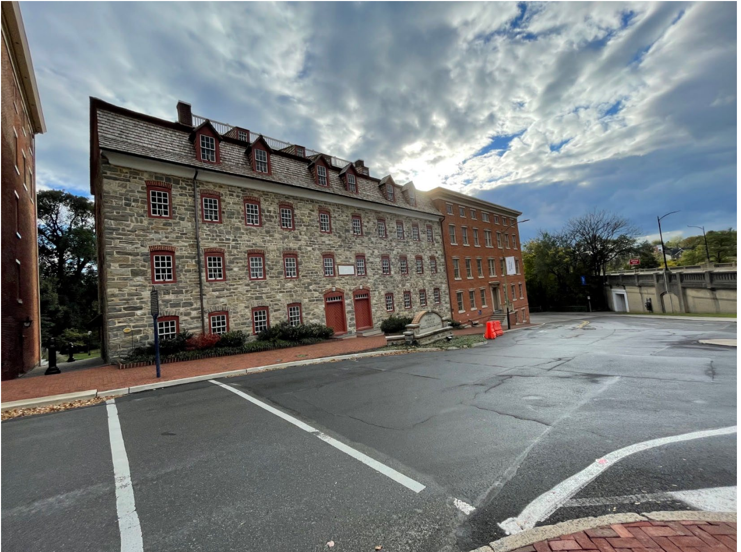
1748 Single Brethren's House Historic Moravian Bethlehem Historic District Front elevation with West Hall addition looking Southwest Photo by Catherine Turton, NPS, 2021
