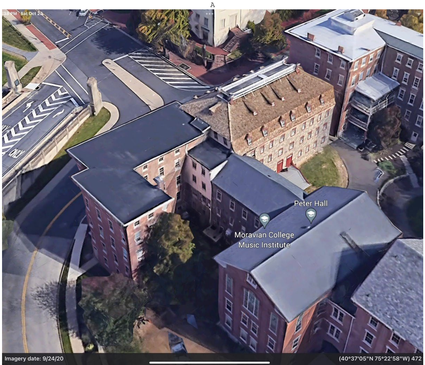
Aerial view of 1748 Single Brethren's House with additions Historic Moravian Bethlehem Historic District Looking Northeast Source: Google Earth
