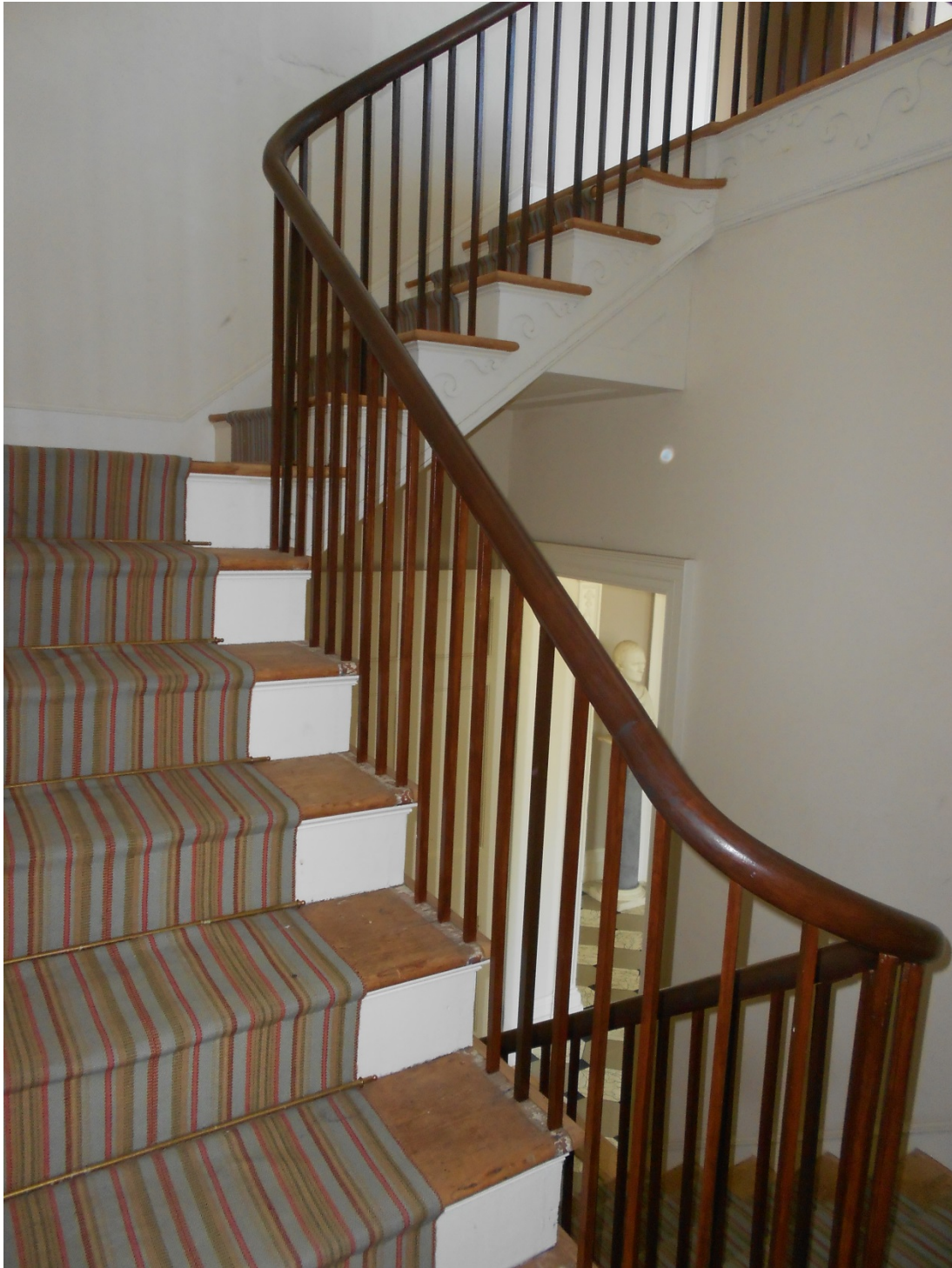
Stairs, camera facing southwest. Caridad de la Vega, photographer, July 22, 2016
