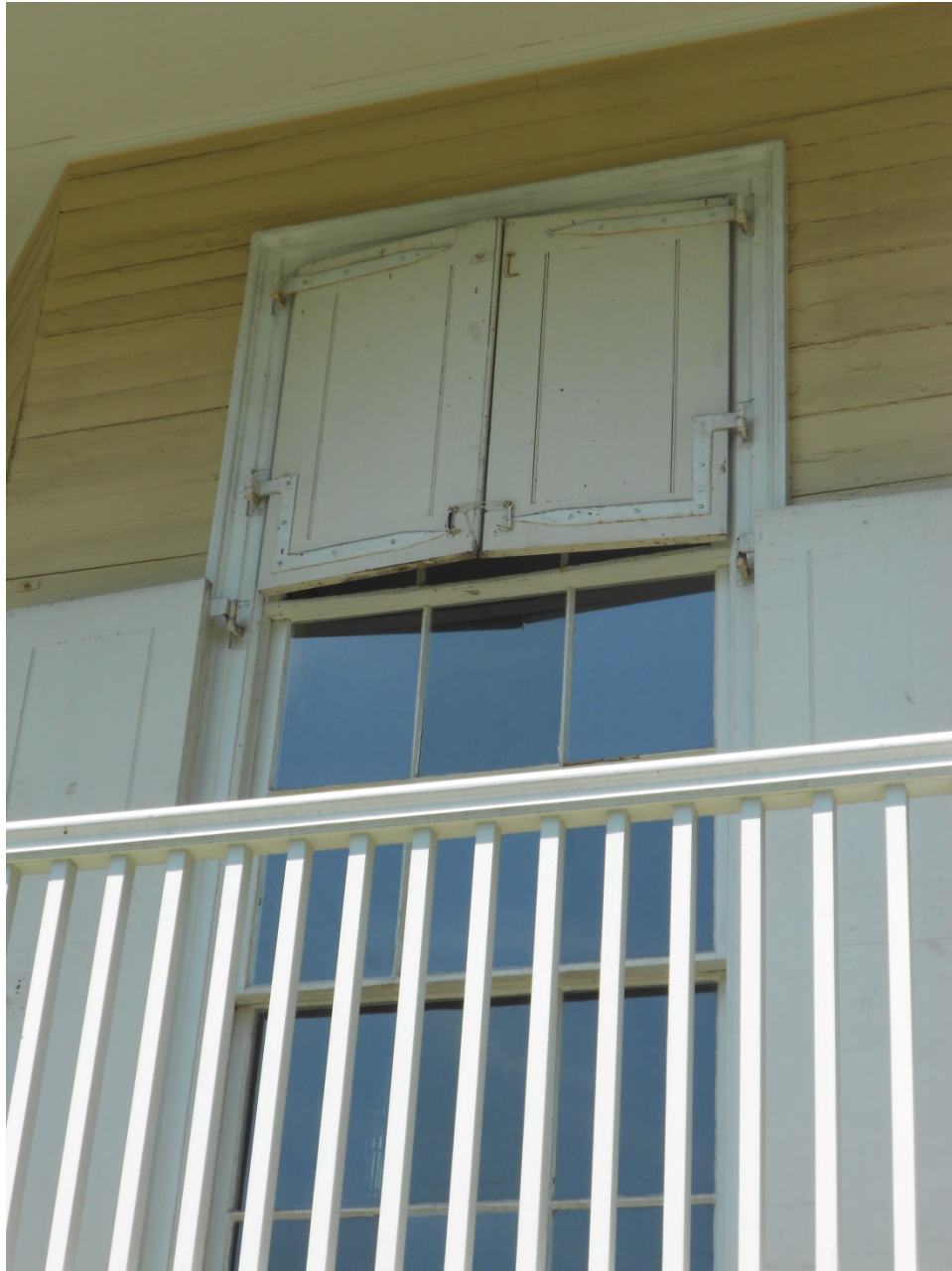
Detail of triple-hung window and shutters on east elevation, camera facing west. Caridad de la Vega, photographer, July 22, 2016
