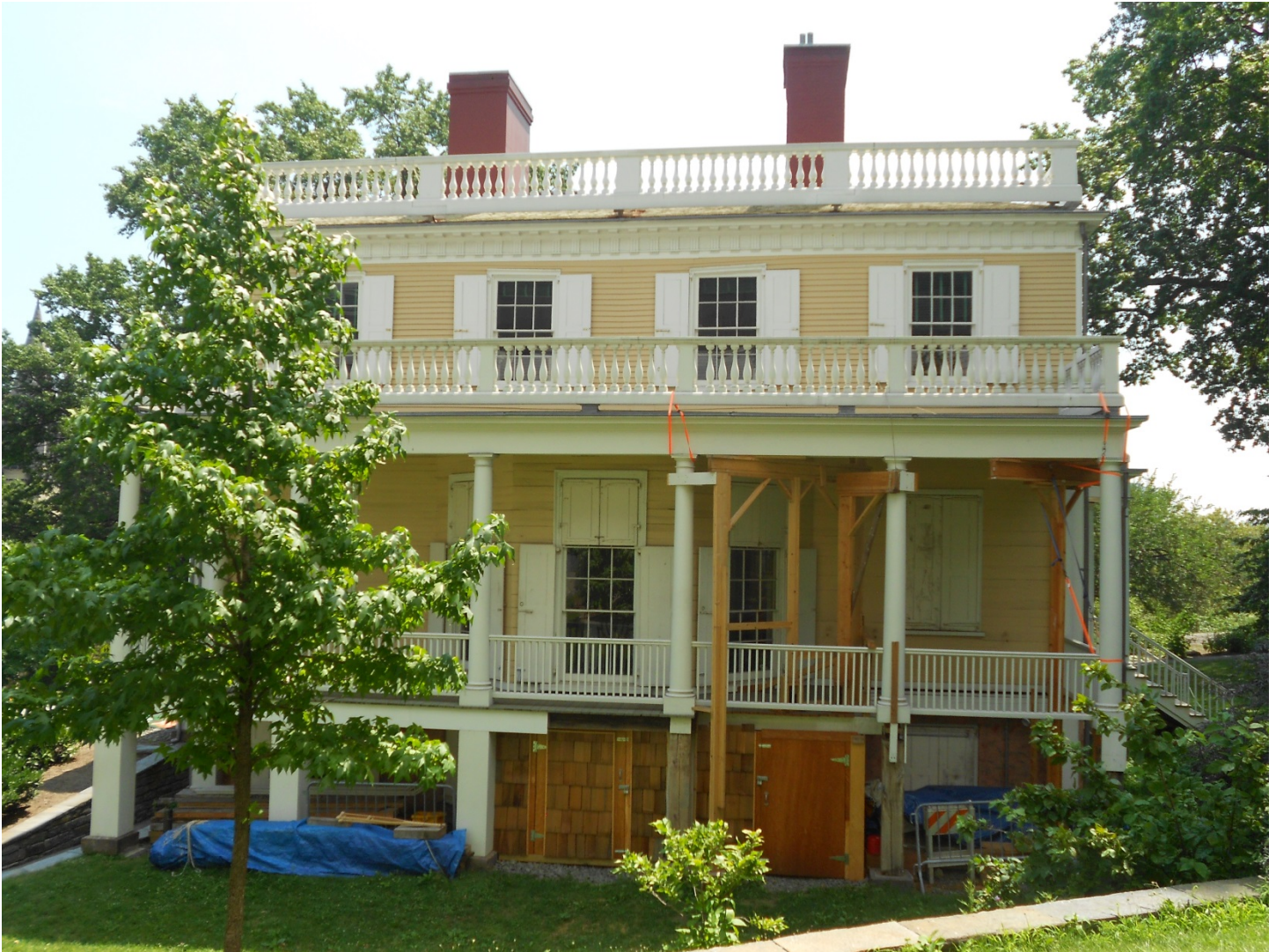
West elevation, camera facing east. Caridad de la Vega, photographer, July 22, 2016
