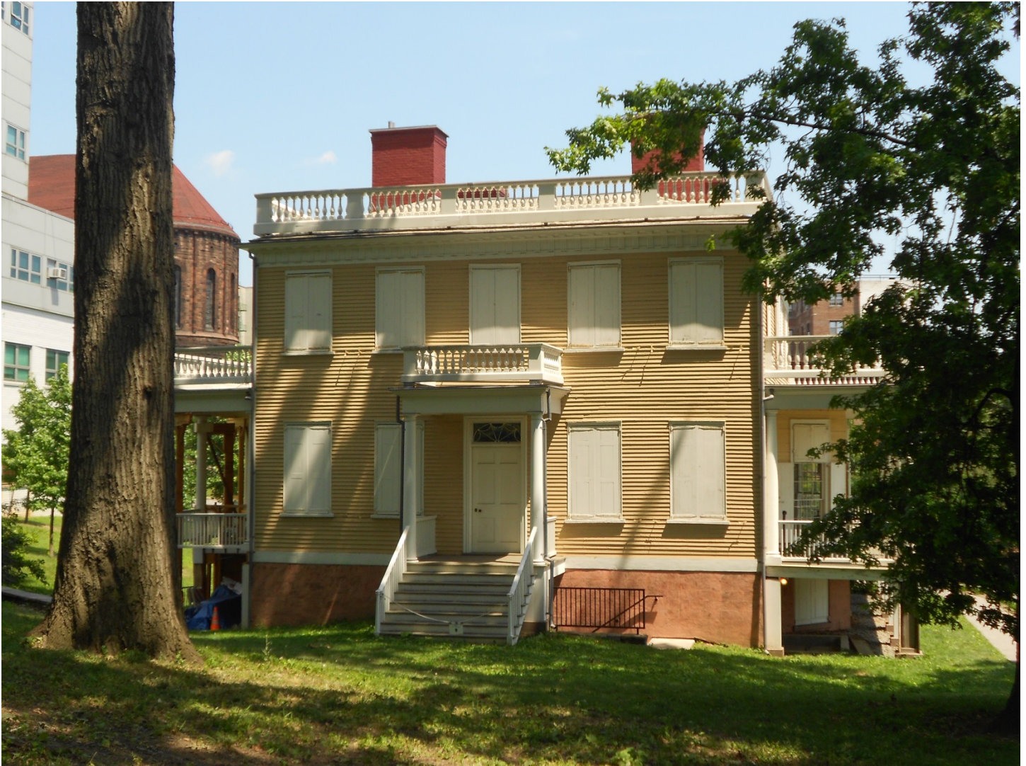
South elevation, camera facing north. Caridad de la Vega, photographer, July 22, 2016
