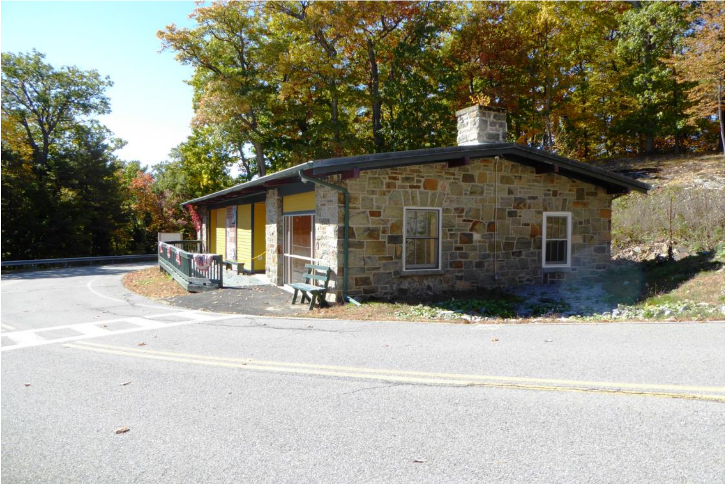
Photo 9: The south and east elevations of the site's visitor center, adapted from a sanitarium-era garage located southeast of Grant Cottage along the approach road, view toward the west.
