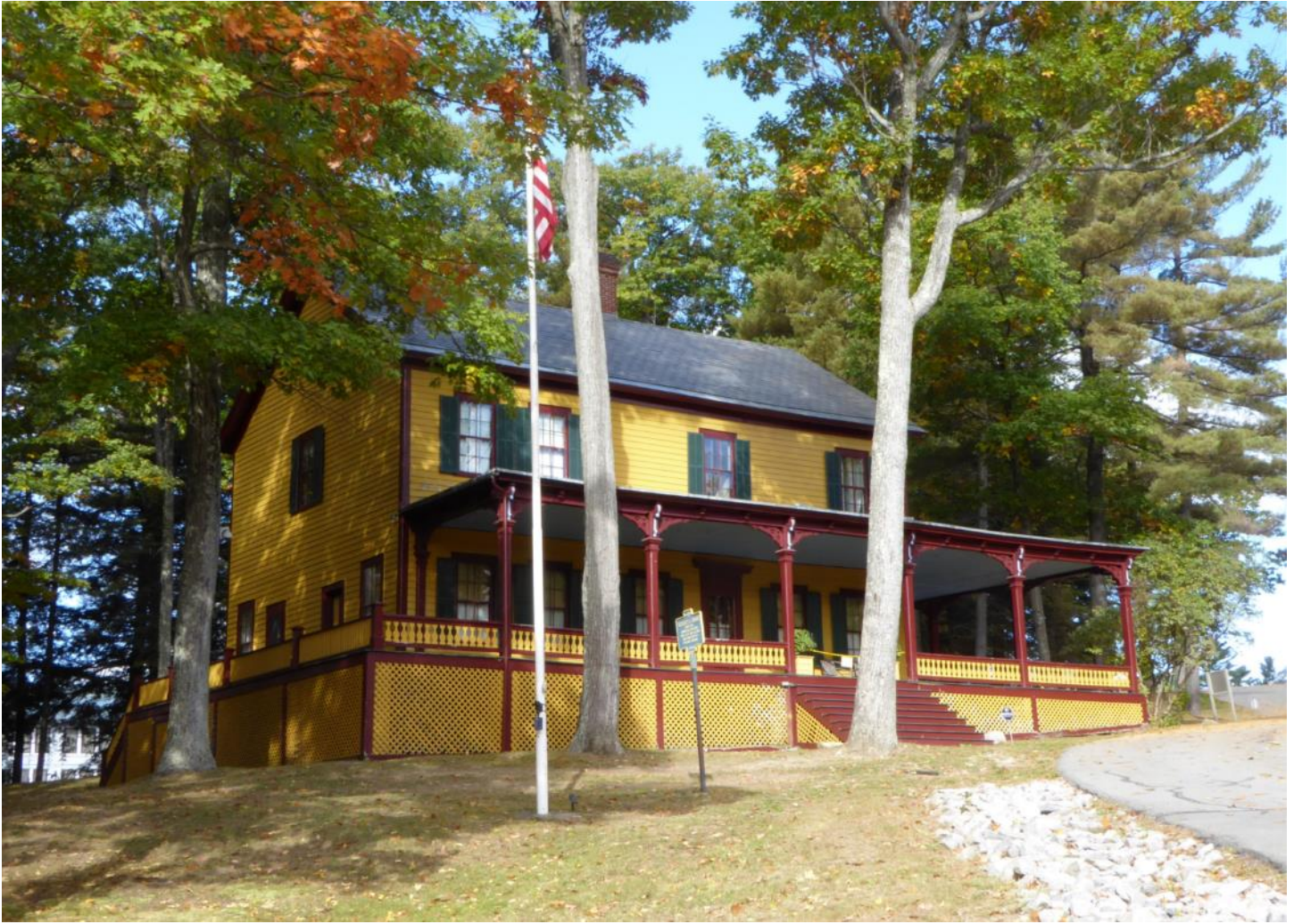
Photo 1: South and east elevations, view toward northwest. Photographer Wes Haynes October 2016
