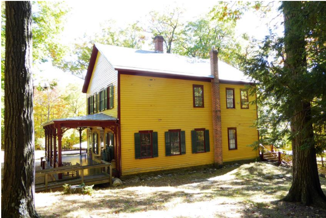
Photo 3: North and west elevations, view toward southeast.
