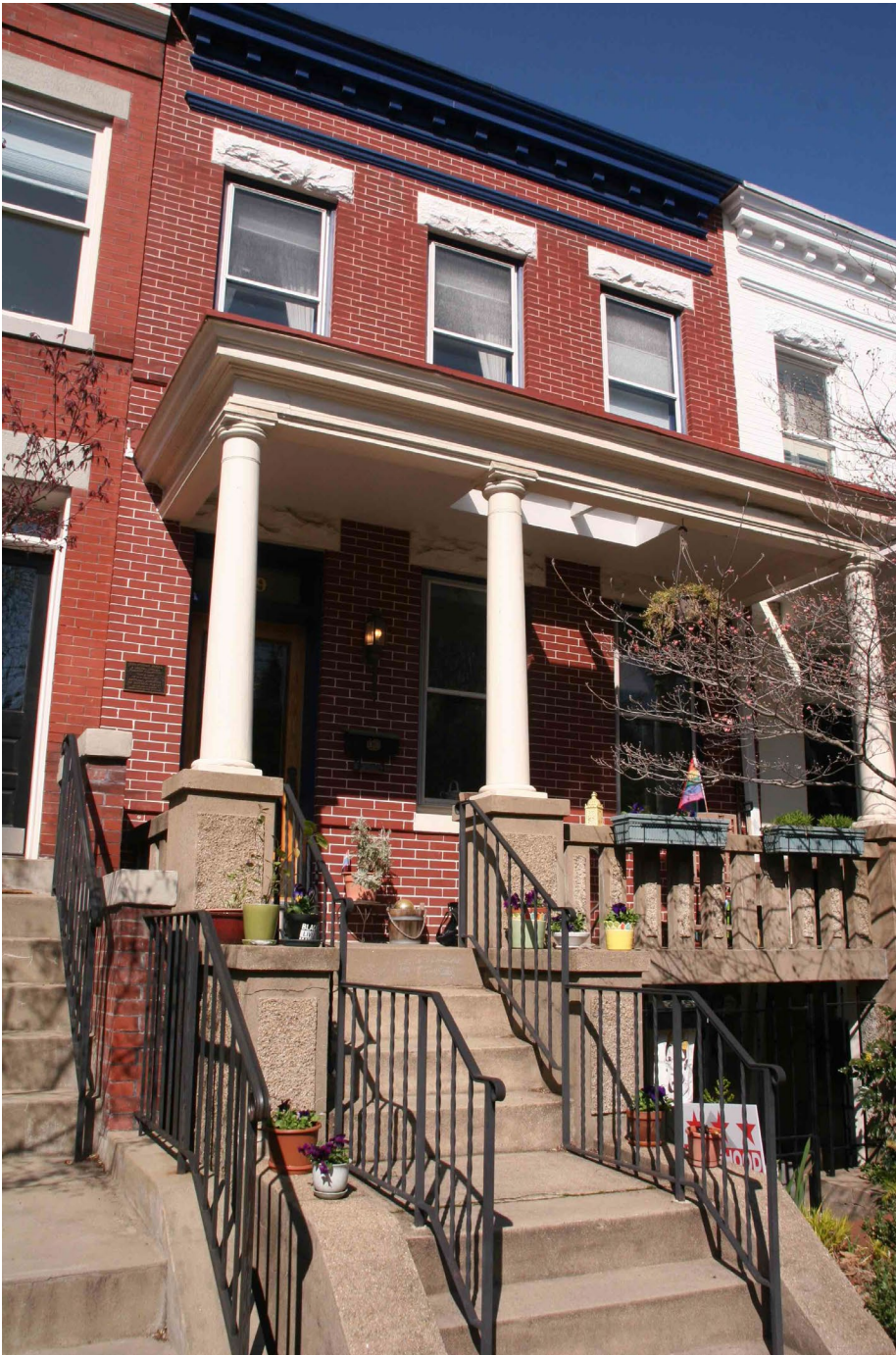
Photo 1 of 10 East Elevation (front). Camera facing west.
