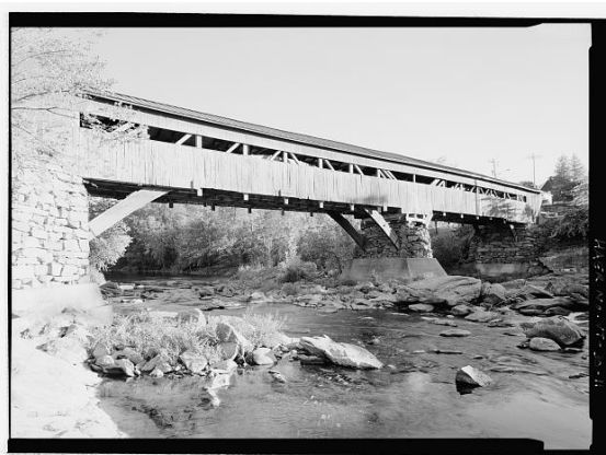
Taftsville Bridge (1836) Taftsville, Windsor County, Vermont Solomon Emmons III, Builder Multiple kingpost truss
