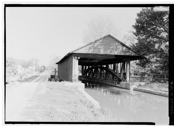
Duck Creek Aqueduct (1848) Metamora, Franklin County, Indiana Whitewater Canal Company, Builder Burr truss
