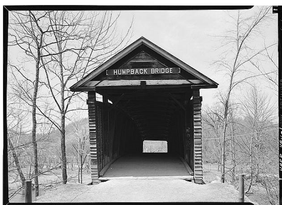
Humpback Bridge (1857) Covington vicinity, Alleghany County, Virginia James River & Kanawha Turnpike Company, Builder Multiple kingpost truss
