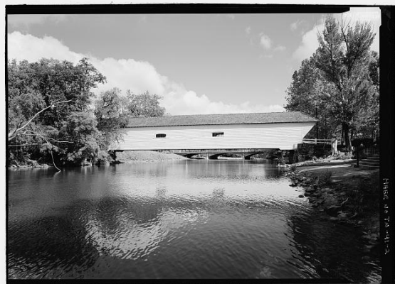
Doe River Bridge (1882) Elizabethton, Carter County, Tennessee Thomas Matson, Engineer E.E. Hunter, General Contractor Howe truss
