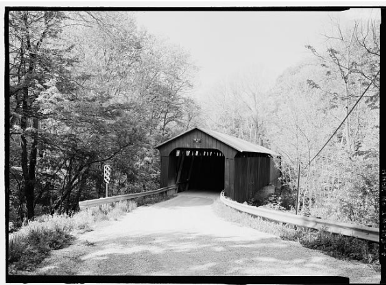
Pine Bluff Bridge (1886) Bainbridge vicinity, Putnam County, Indiana Joseph A. Britton, Builder Howe truss
