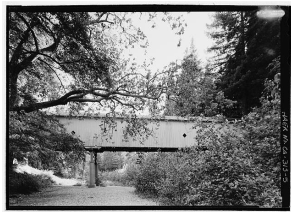
Powder Works Bridge (1872) Santa Cruz, Santa Cruz County, California Pacific Bridge Company, Builder Smith truss
