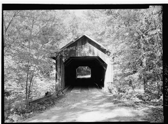
Brown Bridge (1880) Shrewsbury, Rutland County, Vermont Nichols M. Powers, Builder Town lattice truss
