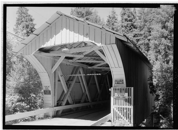
Powder Works Bridge (1872) Santa Cruz, Santa Cruz County, California Pacific Bridge Company, Builder Smith truss
