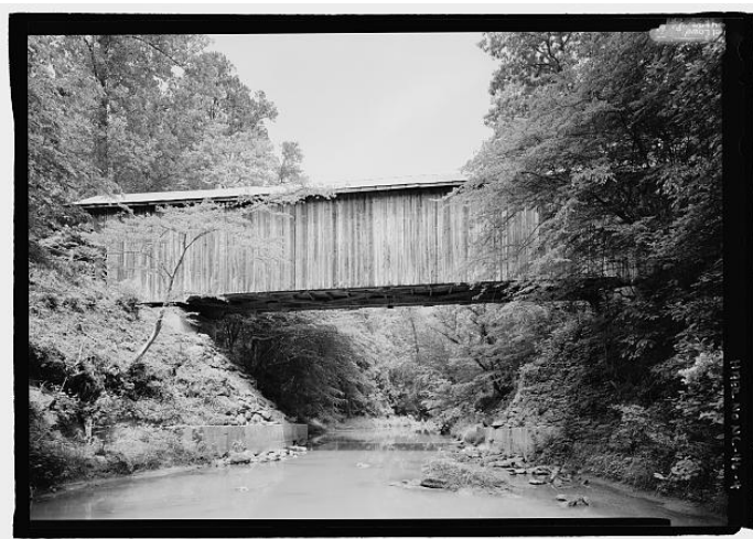
Bunker Hill Bridge (1895) Claremont vicinity, Catawba County, North Carolina Andrew L. Ramsour, Builder Haupt truss
