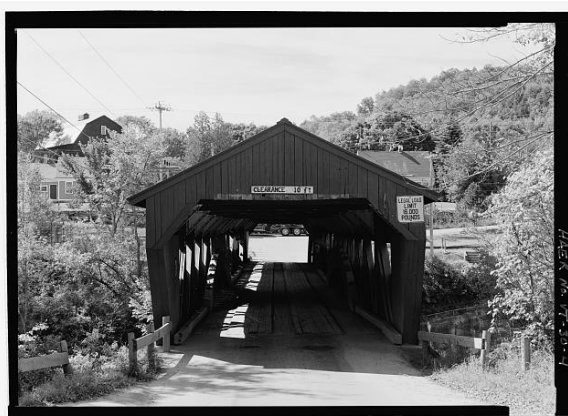
Taftsville Bridge (1836) Taftsville, Windsor County, Vermont Solomon Emmons III, Builder Multiple kingpost truss
