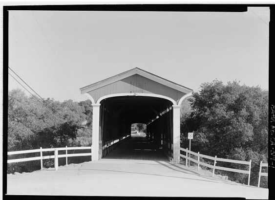
Knight's Ferry Bridge (1863) Knight's Ferry, Stanislaus County, California Schuylkill Construction Company, Builder Howe truss
