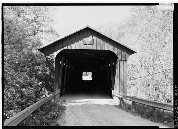
Pine Bluff Bridge (1886) Bainbridge vicinity, Putnam County, Indiana Joseph A. Britton, Builder Howe truss
