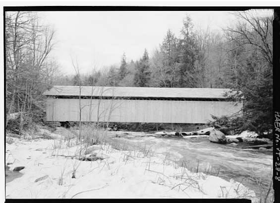
Brown Bridge (1880) Shrewsbury, Rutland County, Vermont Nichols M. Powers, Builder Town lattice truss
