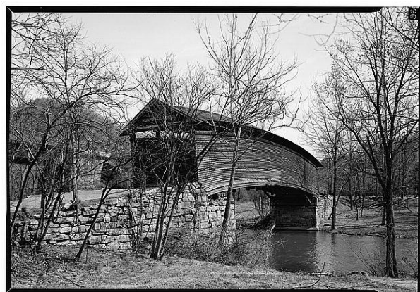
Humpback Bridge (1857) Covington vicinity, Alleghany County, Virginia James River & Kanawha Turnpike Company, Builder Multiple kingpost truss
