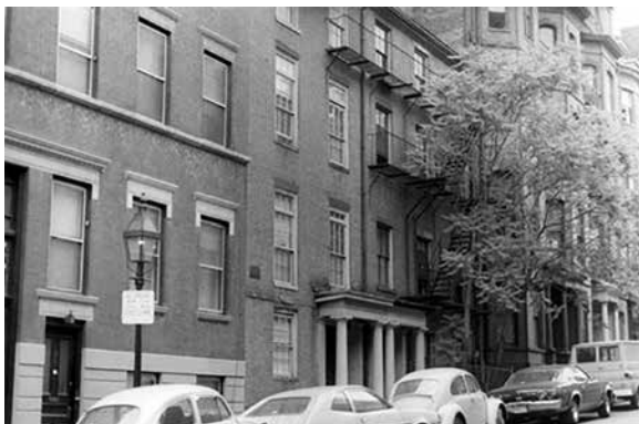
Charles Sumner House, Boston, Massachusetts (National Historic Landmark photograph).
