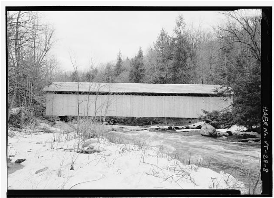
BROWN BRIDGE. View from downstream. Photograph by Jet Lowe, 2003 [HAER VT-28-8]
