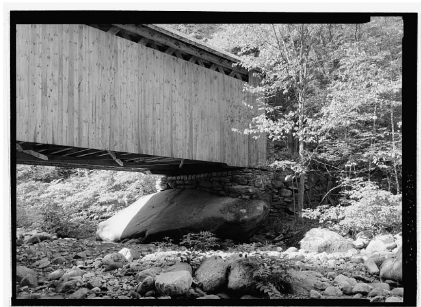
BROWN BRIDGE. Southwest abutment detail from downstream. Photograph by Jet Lowe, 2004 [HAER VT-28-6]
