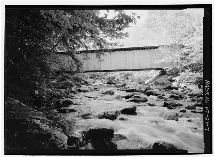
BROWN BRIDGE. View from downstream. Photograph by Jet Lowe, 2004 [HAER VT-28-7]
