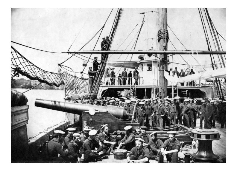
**Figure 15**. A crew prepares to test a 10-inch (25.4-centimeter) caliber, 300-pounder Parrott gun mounted on the West Point Foundry's testing platform (photograph dated May 1, 1864). Nearly two years earlier, President Abraham Lincoln witnessed a similar test conducted from this point. The remains of the testing platform would later be excavated and partly removed under the direction of Joel Grossman in the early 1990s. Courtesy of Putnam History Museum. Used with permission.
