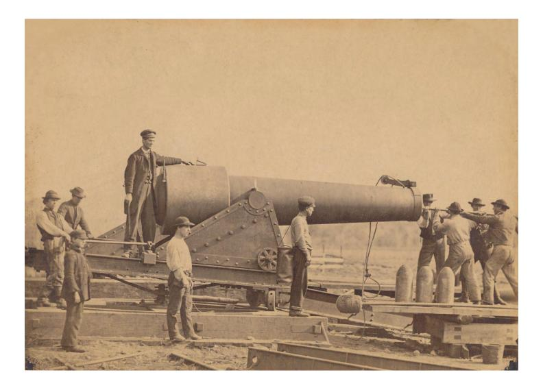
**Figure 16**. A gun crew demonstrates the firing position of an 8-inch (20.3-centimeter) caliber, 200-pounder Parrott gun, mounted in Battery Chatfield and aimed at Fort Sumter in Charleston Harbor. Courtesy of Library of Congress, Prints and Photographs Online Catalog - Civil War.
