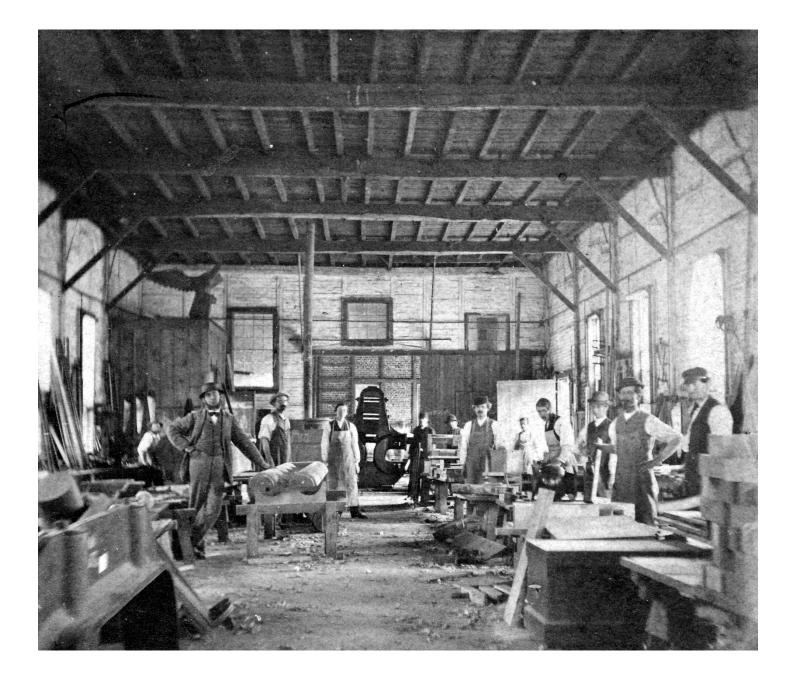
**Figure 11**. An interior view of the machine shop and some of its workers during the Civil War period, with at least two Parrott guns mounted on boring beds in the background. The jib crane visible in the background was used to transfer ordnance pieces between railcars and the boring beds. Courtesy of Putnam History Museum. Used with permission.
