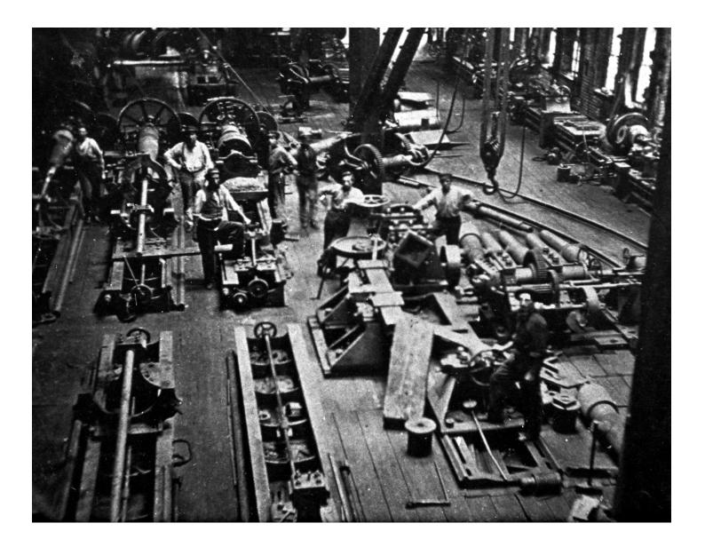
**Figure 12**. An interior view of the blacksmith shop during the Civil War period. Note the finished Parrott gun breech band on the floor in the foreground and three large steam hammers in the background. The largest of the three steam hammers is likely depicted in John Ferguson Weir's painting *Forging the Shaft* (see Figure 21). Courtesy of Putnam History Museum. Used with permission.
