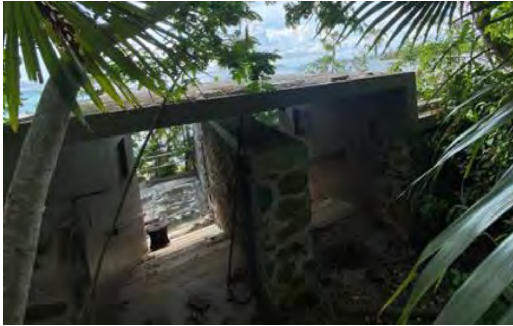
Figure 5 – Flat Roof over Breezeway Stairs
