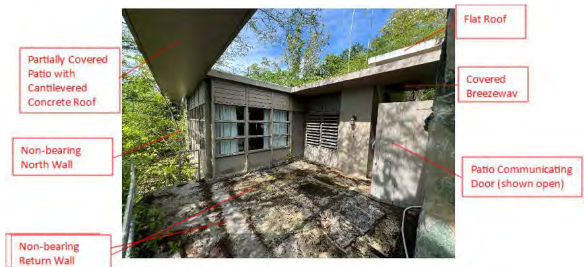
Figure 3 - Exterior Cottage View with Labels
