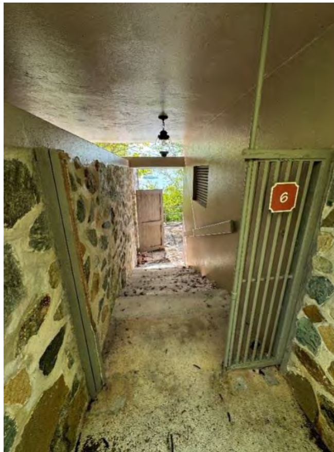
Figure 1 - Breezeway Stair to Cottage Entrance
