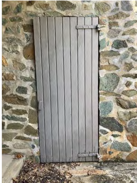
Figure 4 – Patio Communicating Door
