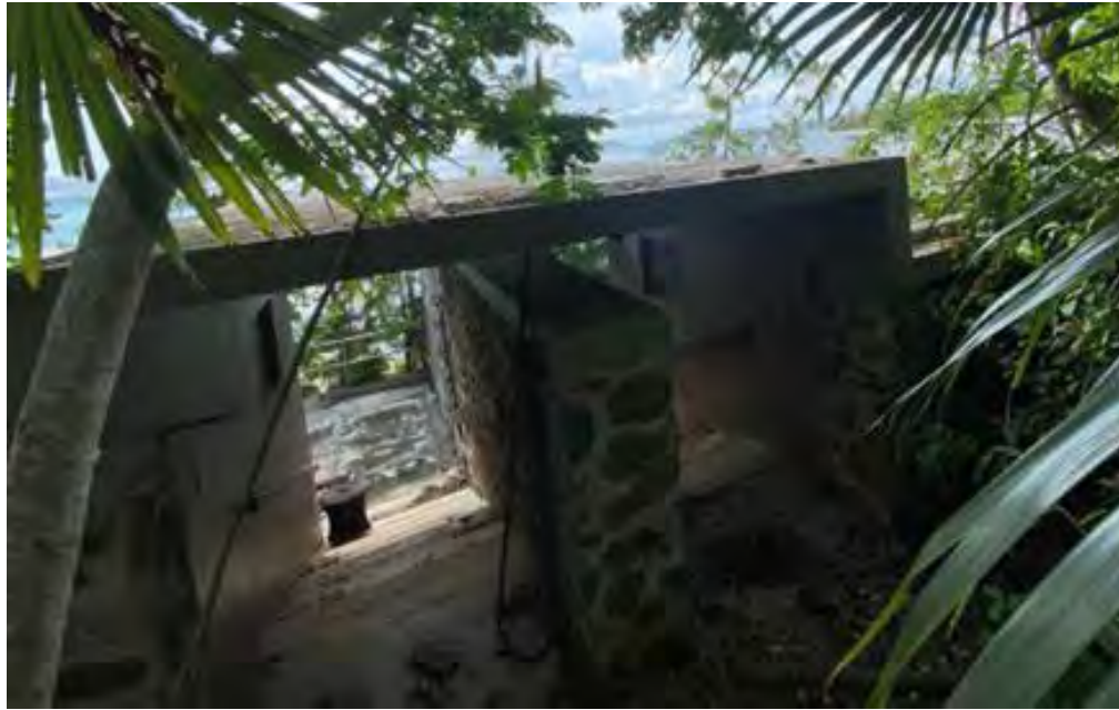
Figure 5 – Flat Roof over Breezeway Stairs
