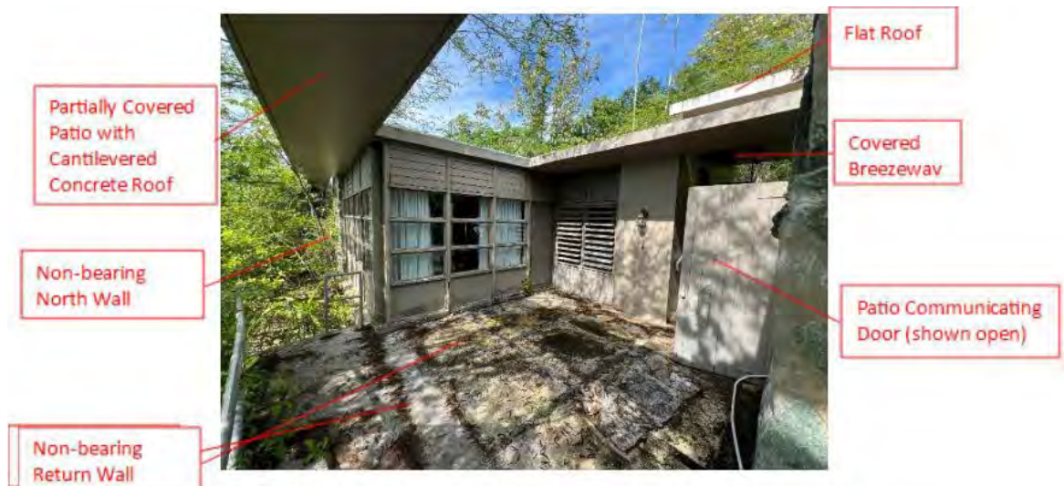
Figure 3 - Exterior Cottage View with Labels
