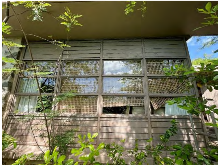
Figure 6 – North Facing Non-Load Bearing Walls
