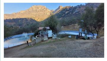
The project focuses on rehabilitating and replacing critical components. It includes two pump stations and controls, the associated signage, fencing, access road, and electrical and monitoring systems. The project also addresses deteriorated headworks, overflow, chlorination system, treatment dosing building, and disposal fields. With 1.2 million annual visitors, the project ensures sustainable wastewater treatment capacity for the Ash Mountain Historic District and supports park employees.
