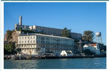
The project aims to address deterioration and structural deficiencies of the Alcatraz Main Prison Building, focusing on the Hospital Wing and exterior walls. It involves abating hazardous materials, repairing concrete spalls, reinforcing deteriorated steel, strengthening foundation walls, stabilizing windows, applying coatings, and matching finishes. The project aims to enhance visitor and staff safety, improve seismic resilience, and mitigate aging and weather-related impacts.
