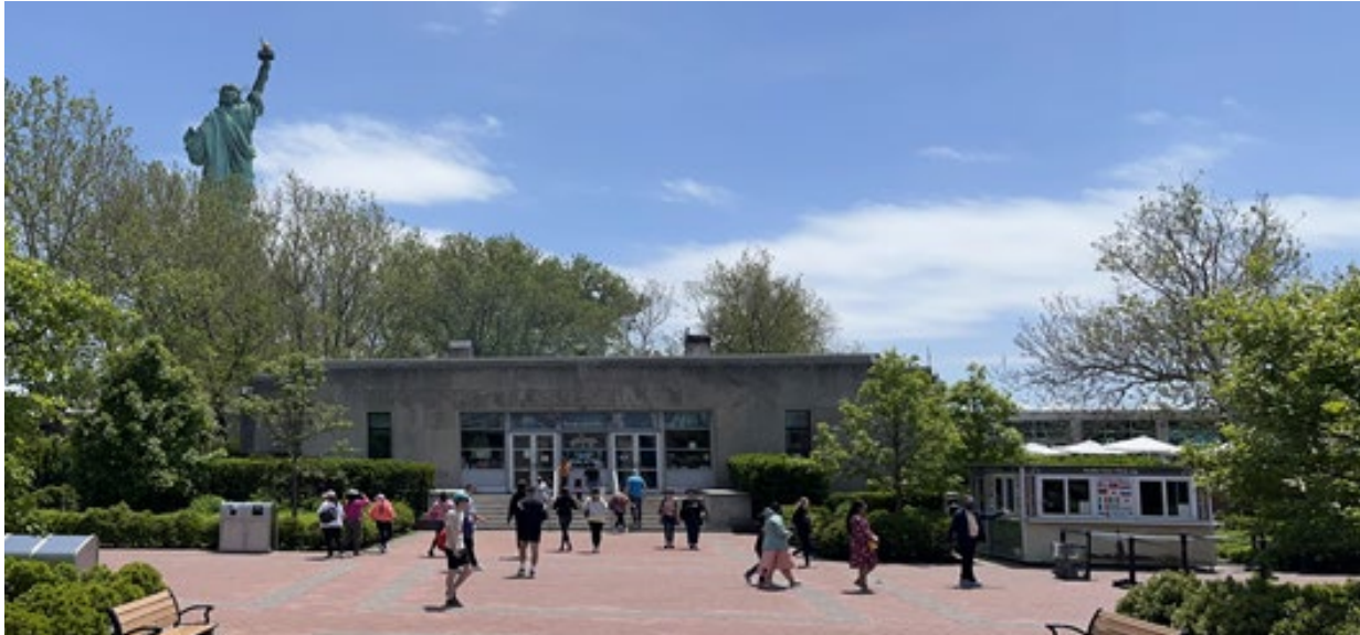
Pictured: Liberty Island Concession Building
