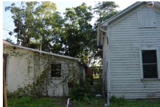
Auxiliary Building South
