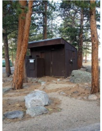
Firewood sales area at Moraine Park Campground
