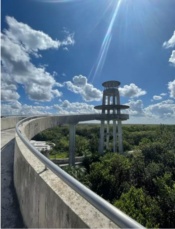
The iconic Shark Valley Tower is a Mission 66 Historic Structure.
