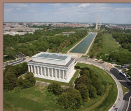
To reduce energy use associated with water treatment, the NPS recently renovated the largest reflection pool at the National Mall and Memorial Parks in Washington D.C. The pool now recirculates water from the nearby Tidal Basin.
