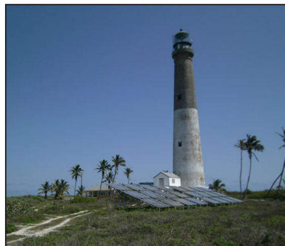
Solar arrays power the generators at Loggerhead Key. NPS Photo
