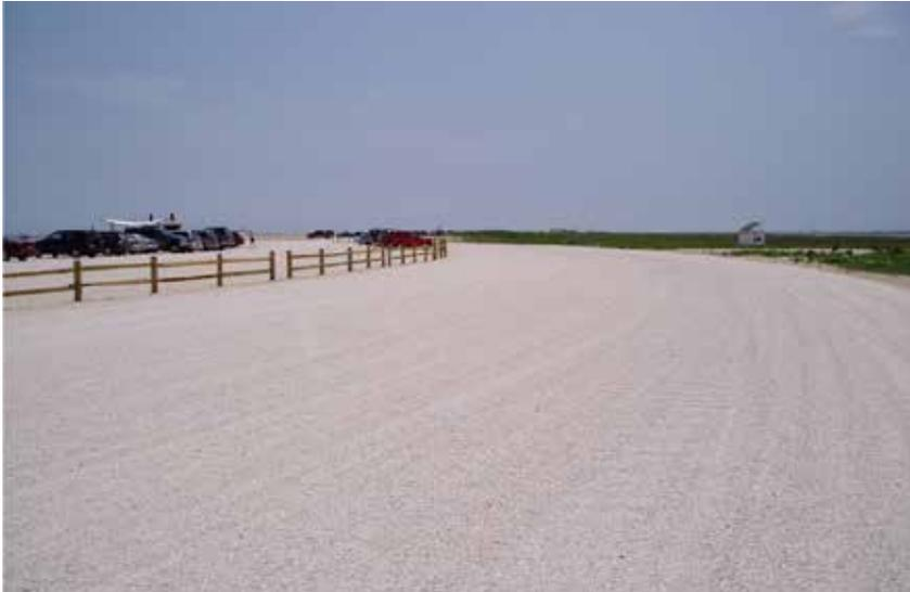
The Virginia visitor parking lot is constructed with native materials including clay and clamshell that can be reused in post-storm repairs. Image credit: Ish Ennis, NPS.
