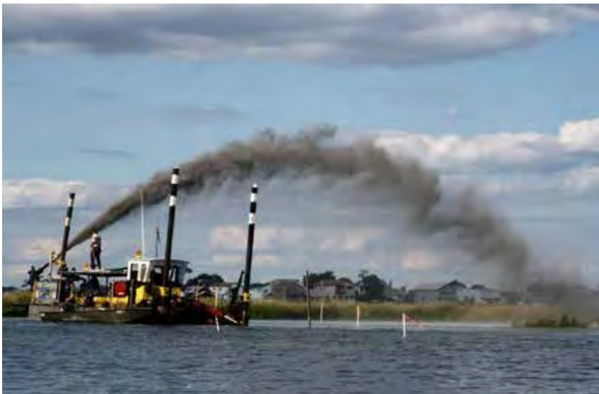
Salt marsh restoration in Jamaica Bay has tried a variety of experimental techniques to increase marsh elevation, including spraying the marsh surface using a swing-ladder dredge. Image credit: USACE New York District.
