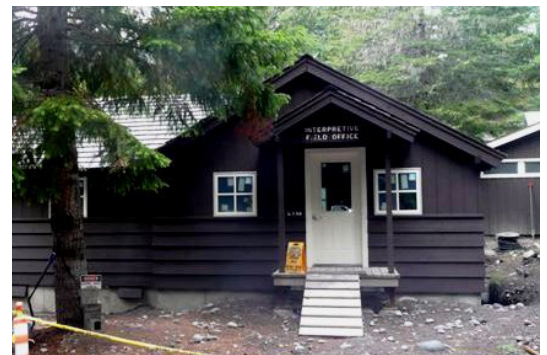
This historic Mt. Rainier office building is nearly identical to the original after Passive House renovations. A couple of subtle differences include the new concrete foundation with crawl space vents, and new energy-efficient casement windows.
