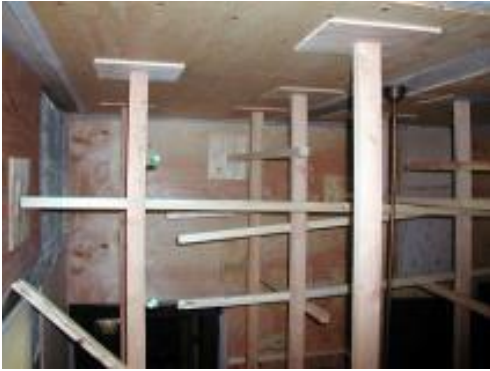
Stabilizing efforts inside the Harada House in 2005
