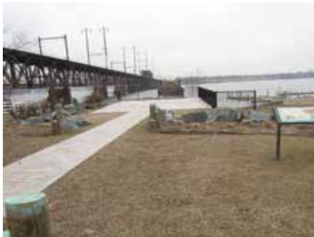
Top: Fishing pier at Pequea, PA (NPS Chesapeake)
