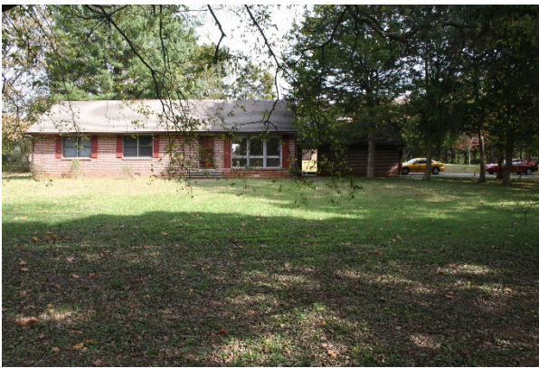
FIGURE 109. Front view of Building 6, looking north. Source: Stones River National Battlefield, photo by park staff, 2014.
