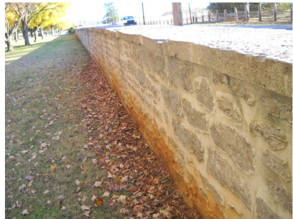
FIGURE B-9, left. Failing mortar joints at the street-facing portion of the site wall.
