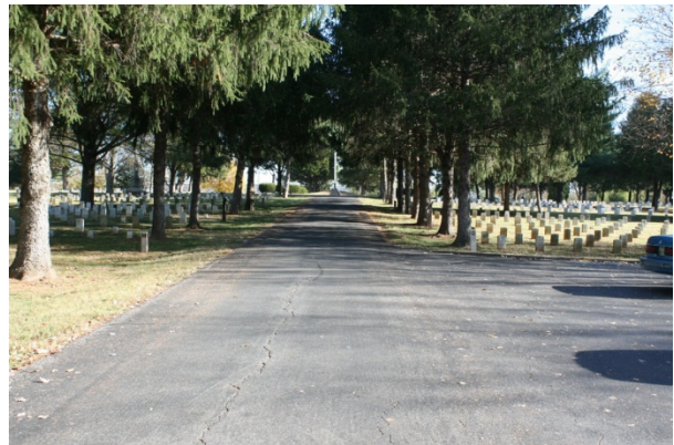
FIGURE 78. The entrance drive extends north from Old Nashville Highway to Lincoln Square. The cannonball pyramid and the flagstaff are visible on axis with the drive.
