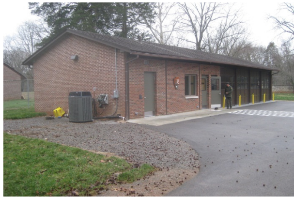
FIGURE 115. The maintenance office and shop building, view from the northeast. Source: Stones River National Battlefield, photo by park staff, 2012.
