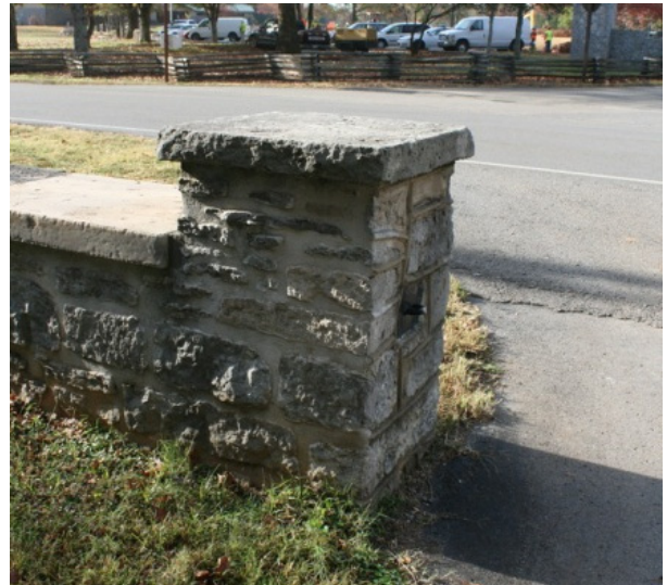
FIGURE 125. A sliding metal pole that extends from the west pier of the gate at the maintenance access drive hooks onto the metal loop of the pier as shown to close this road to public access.
