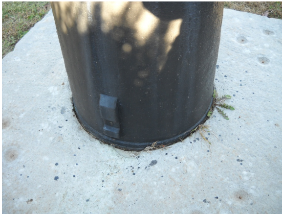
FIGURE B-38. Plant growth in open joint at the base of an upright cannon.
