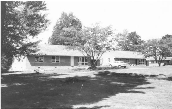
FIGURE 184. The new staff residences under construction, September 1962. The maintenance office and shop building is visible beyond, at right in this view. Source: Stones River National Battlefield Archives, image STRI-Central Files 679.
