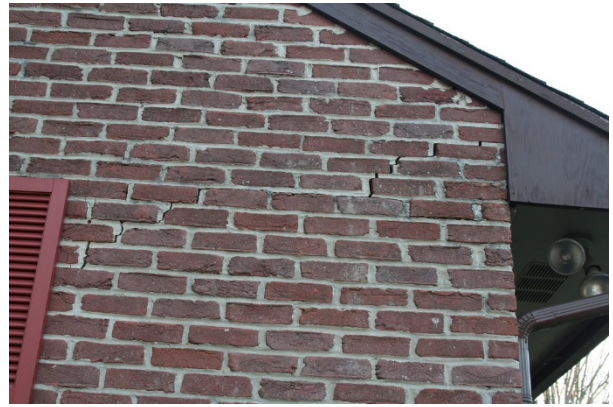
FIGURE 111. Cracked brick masonry is evident near the roof of Building 6. Source: Stones River National Battlefield, photo by park staff, 2014.
