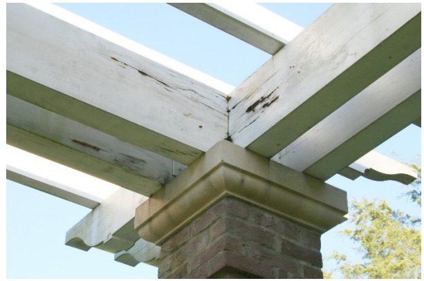
FIGURE 101. Deterioration of wood trellis. Source: Stones River National Battlefield, photo by park staff, 2014.
