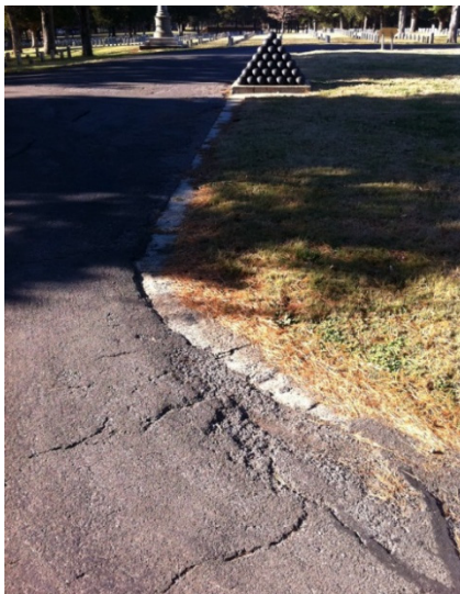
FIGURE 81. Concrete curbing along Central Avenue as it loops around Lincoln Square. Also visible is the cracked asphalt pavement of the road.
