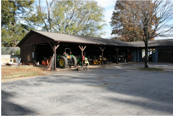
FIGURE 117. The garage is an open structure used to store equipment.
