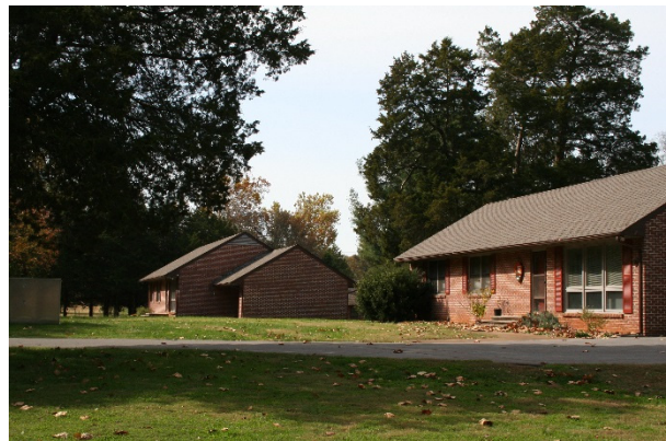
FIGURE 107. View looking south of Building 4 (at right) and Building 5 beyond (at left). Source: Stones River National Battlefield, photo by park staff, 2014.
