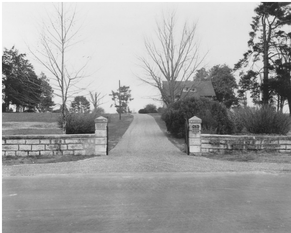
FIGURE 194. The completed maintenance gate, March 1938. Source: Stones River National Battlefield Archives, image STRI-ICP-0440.
