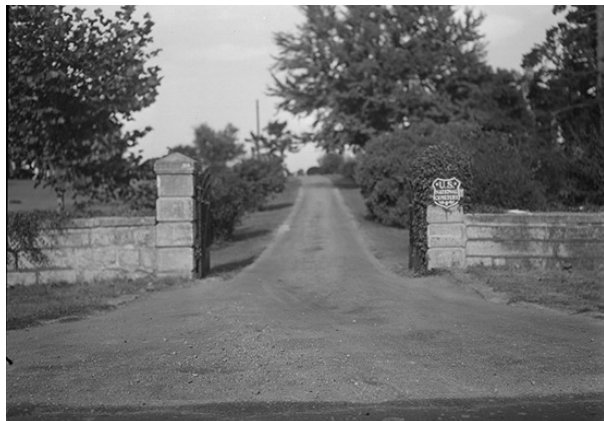
FIGURE 25. An undated view of main entrance gate; the 1913 iron shield is visible on the right pier. Source: Stones River National Battlefield Archives, image STRI-NN-0166. Note the rusticated concrete piers constructed in 1896.
