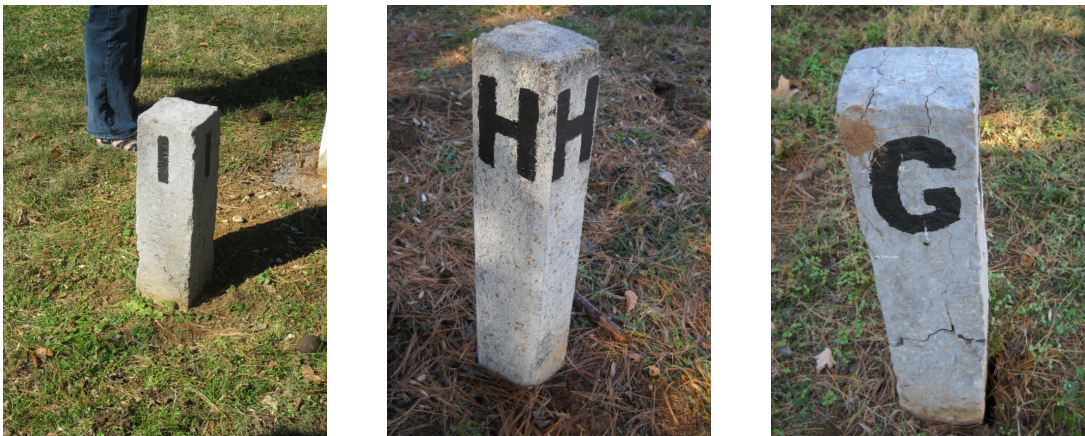
FIGURE B-28, left. Example of limestone section marker with chipping at the corners.
