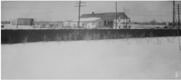
FIGURE 33. Cemetery wall looking west across Old Nashville Highway, after screen planting. Source: National Archives, R.G. 79, Records of the Branch of Engineering: Final Construction Reports, Box 1, Entry 75, Superintendent Richard B. Rudolph, "Report on Plating at Stones River National Military Park: Public Works Project No. 481" (February 6, 1935.)
