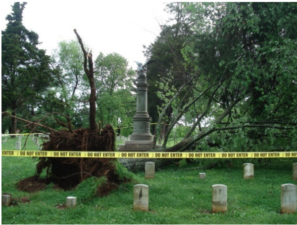
FIGURE 49. The U.S. Regulars Monument narrowly escaped damage when a nearby tree was uprooted by a tornado. Source: Stones River National Battlefield, photo by park staff.
