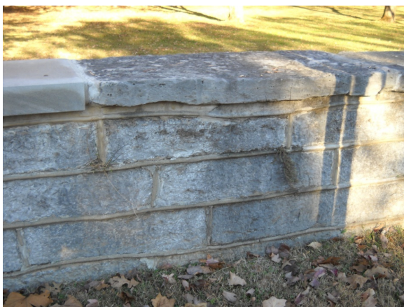
FIGURE B-11, left. Plant growth at mortar joints.
