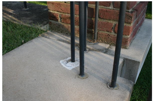
FIGURE 103. Previous patching and sealant failure at embedded railing post. Source: Stones River National Battlefield, photo by park staff, 2014.
