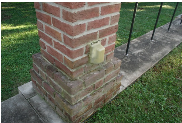
FIGURE 100. Detail of moisture-related staining at the base of the brick posts. Source: Stones River National Battlefield, photo by park staff, 2014.
