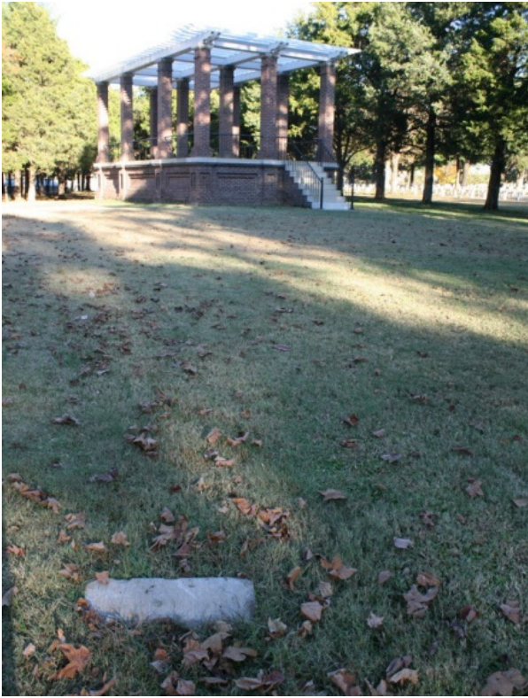
FIGURE 154. A concrete storm water outfall is located near the rostrum and is associated with draining the earthen base of the structure.
