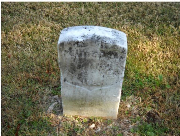
FIGURE B-25, left. Erosion and surface wear of inscribed shield and projecting lettering on Civil War era grave marker.
