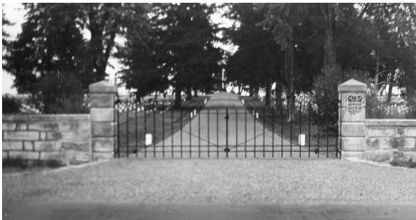
FIGURE 189. The completed main entrance gate, circa 1937. Note the freshly repointed joints in the limestone wall adjacent to each pier, indicating the extent of the wall affected by the 1930s work. Source: Stones River National Battlefield Archives, image STRI-ICP-0405.
