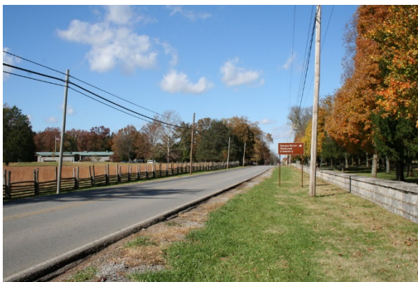
FIGURE 140. Overview of directional signage along Old Nashville Highway. Source: Stones River National Battlefield, photo by park staff, 2014.
