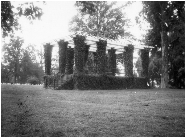
FIGURE 177. The rostrum, circa 1930, view looking southeast. Note the location of the stairs on the western half of the structure's north end. Source: Stones River National Battlefield Archives, image STRI-4X5P-1088.
