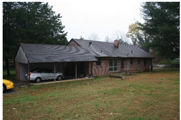
FIGURE 112. A low stone retaining wall is located behind Building 6. It was built around a tree that has since been lost. Source: Stones River National Battlefield, photo by park staff, 2014.
