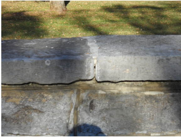
FIGURE B-7, left. View of coping stones and wall field stone.
