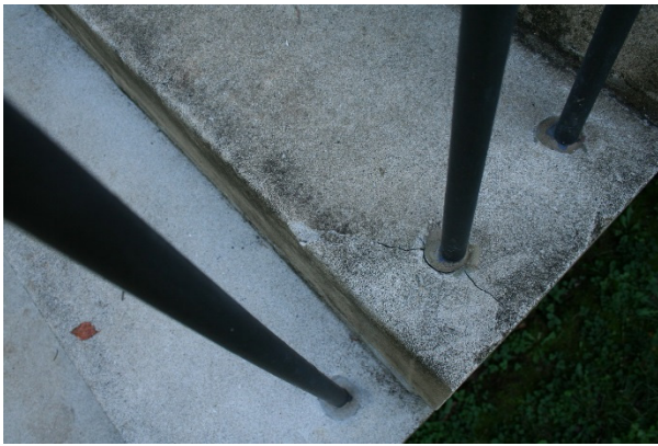
FIGURE 104. Cracking of stair tread at embedded railing post. Source: Stones River National Battlefield, photo by park staff, 2014.
