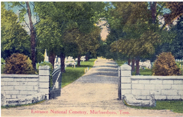
FIGURE 187. Postcard view of the main gate, circa 1910, showing rusticated concrete piers constructed in 1896. This view predates the addition of a cast iron plaque to the east pier in 1913. Note raised stone curbs adjacent to the drive. Source: Stones River National Battlefield Archives, image STRI 4735.
