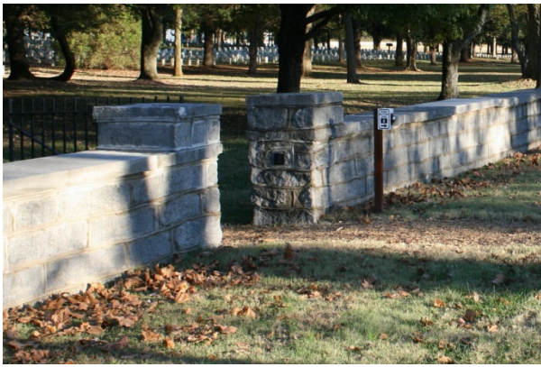
FIGURE 196. The reconstructed pedestrian gate, 2010, seen from the opposite angle. The piers as constructed are different from those shown above circa 1930s, with the cap at the top of the wall extending through the pier rather than stopping at the pier face.
