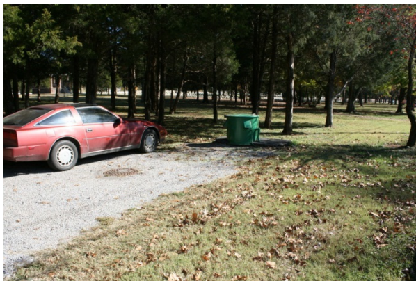
FIGURE 88. A gravel access road leads from the maintenance access drive to the sewer pump station, shown with a green cover, located inside the cemetery.
