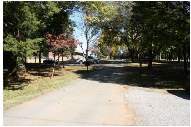
FIGURE 89. The access drive extends in a north/south direction through the lodge and service area.
