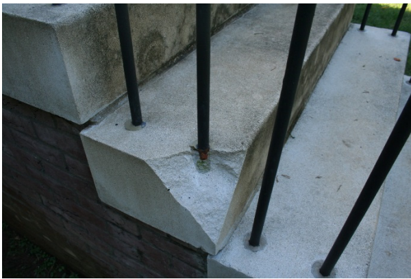
FIGURE 105. Spalled cast stone stair tread at embedded railing post. Source: Stones River National Battlefield, photo by park staff, 2014.
