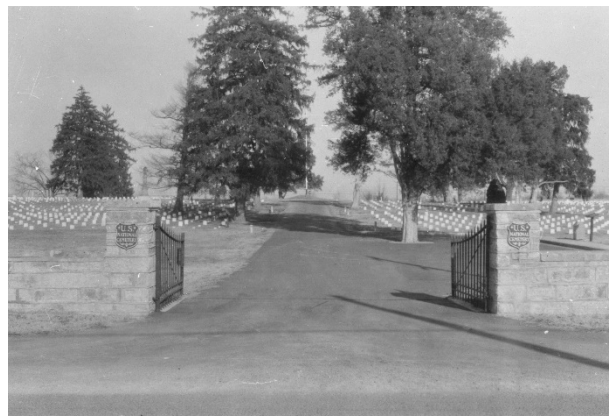
FIGURE 190. The reconstructed main entrance gate, circa 1961–1963. The cast metal plaque at the service entrance was moved to the west pier of the main entrance. The 1937 cast iron gates were repaired and reinstalled. Source: Stones River National Battlefield Archives, image STRI-Central Files 516.
