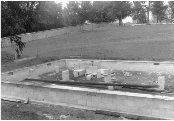
FIGURE 183. View of foundation construction for Quarters 6, June 1962. The former site of the stable is beyond, where disturbed earth is visible. The well house is visible at upper right in this view. Source: Stones River National Battlefield Archives, image STRI-ICP-1208.
