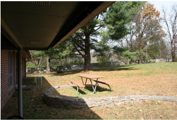
FIGURE 70. Stone retaining wall behind Building 6. Source: Stones River National Battlefield, photo by park staff, 2014.
