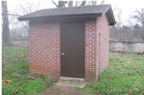
FIGURE 116. The well house.
