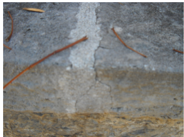
FIGURE B-9, left. Failing mortar joints at the street-facing portion of the site wall.
