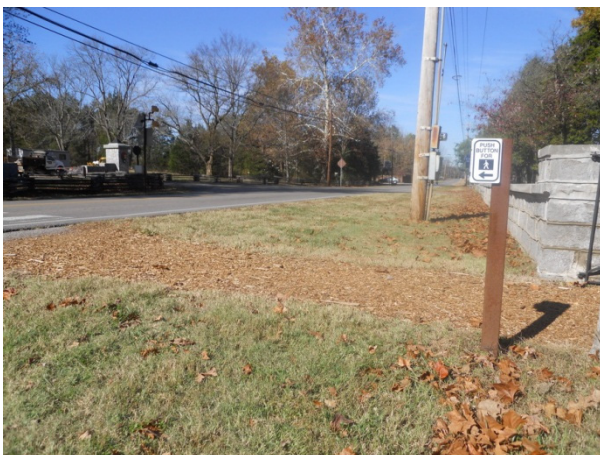
FIGURE 85. A push-button pedestrian crossing warning light system is used to support the safety of pedestrians crossing Old Nashville Highway.
