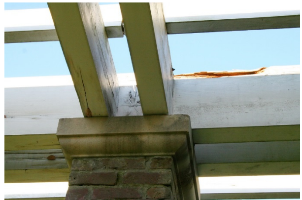
FIGURE 102. Splitting and staining of wood trellis. Source: Stones River National Battlefield, photo by park staff, 2014.
