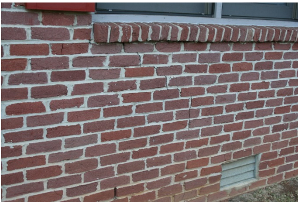
FIGURE 110. Cracked brick masonry, Building 6. Source: Stones River National Battlefield, photo by park staff, 2014.
