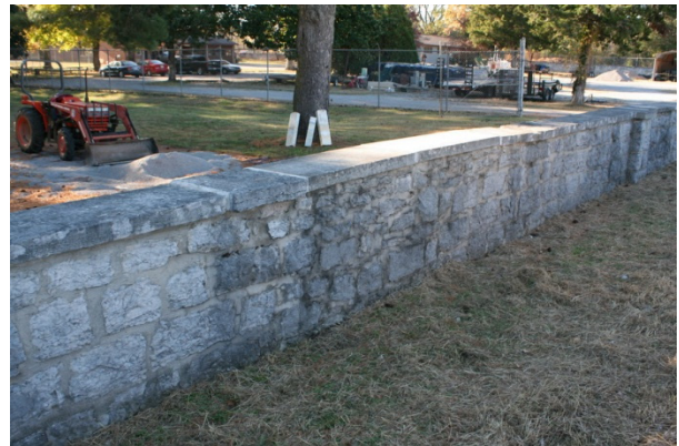
FIGURE 90. A pedestrian entrance associated with rail access was closed in 1963 when passenger service was discontinued. It is likely that the variations in stone and mortar in the section of the wall shown here indicate the location of the former entrance.
