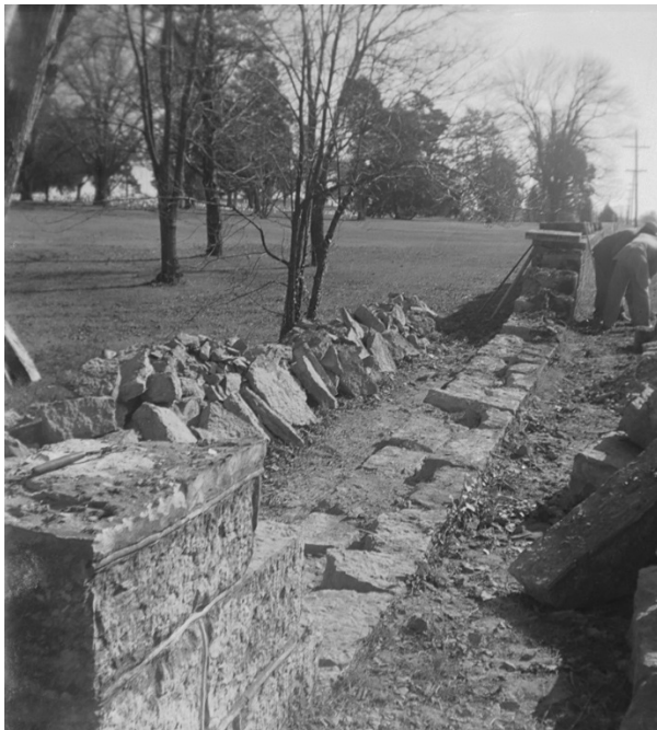
FIGURE 175. Reconstruction of a portion of the perimeter wall, circa 1930s. Source: Stones River National Battlefield Archives, image STRI-AN-035b.
