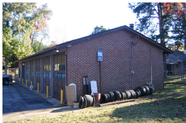
FIGURE 52. The maintenance shop before renovation, view from the northwest, November 2010.
