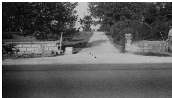
FIGURE 31. The maintenance gateway undergoing reconstruction, 1937. Source: National Archives, Record Group 79: Records of the National Park Service, Records of the Branch of Engineering, Final Construction Reports, 1934–1942.
