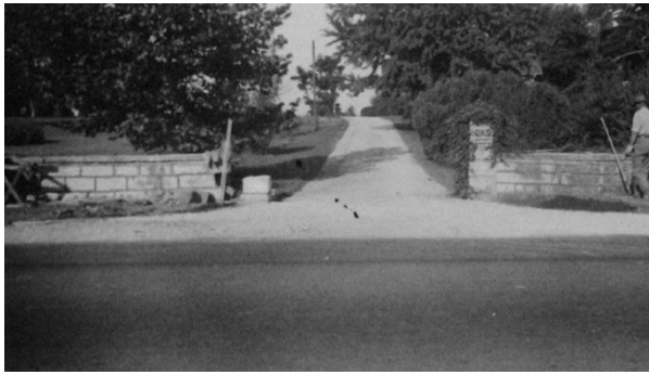
FIGURE 193. The service gateway undergoing reconstruction, 1937. Source: National Archives, Record Group 79: Records of the National Park Service, Records of the Branch of Engineering, Final Construction Reports, 1934–1942.
