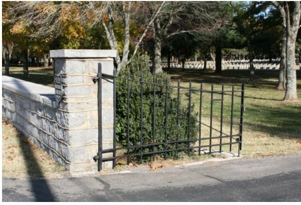
FIGURE 123. The main entrance gate is double-hung, and composed of wrought iron. Each side swings inward on hinges attached to the stone piers.
