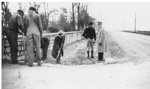
FIGURE 28. The start of drainage work at the north entrance gate to the cemetery in spring 1934. Source: Stones River National Battlefield Archives, image STRI-ICP-0436.
