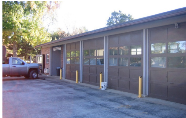
FIGURE 51. The maintenance shop before renovation, view toward the east end of the north elevation, November 2010.
