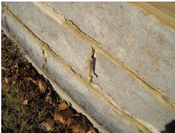
FIGURE B-9, left. Failing mortar joints at the street-facing portion of the site wall.
