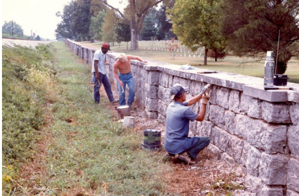
FIGURE 174. Repointing the perimeter wall along the railroad, circa 1980s. Source: Stones River National Battlefield Archives, image STRI-4X5P-1307.
