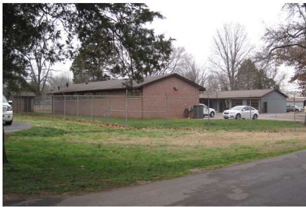
FIGURE 113. View of the maintenance area buildings from the south, including the maintenance office and shop at center, the well house at left, and the storage shed and garage at right. Source: Stones River National Battlefield, photo by park staff, 2012.
