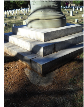
FIGURE B-32, center. Discolored previously placed stone patching material at the U.S. Regulars Monument.
