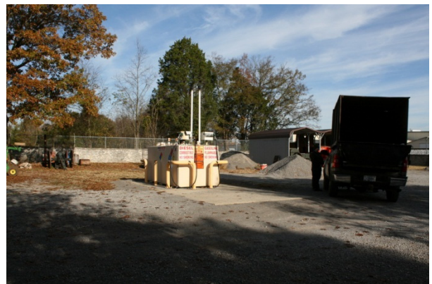
FIGURE 121. The fuel tank located within the maintenance yard.
