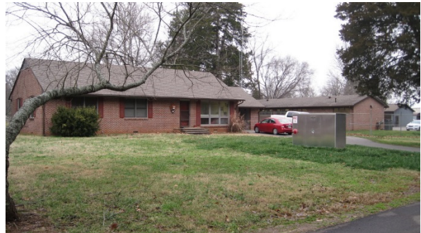
FIGURE 153. A fire department connection box is located on the lawn in front of Building 4 within the staff housing area. Source: Stones River National Battlefield, photo by park staff, 2014.
