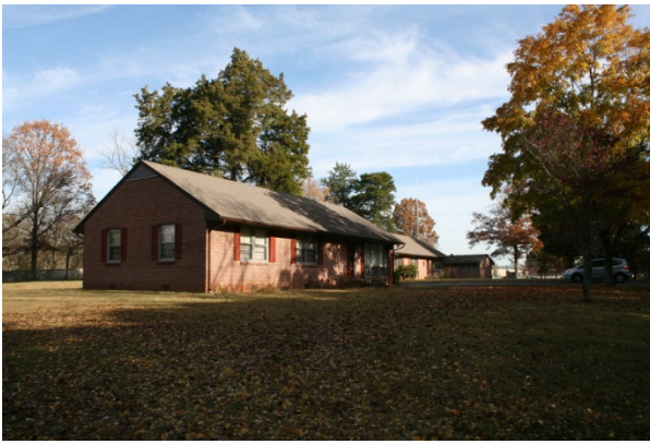
FIGURE 108. Building 5 was constructed in the 1960s and is used by park staff for housing. Source: Stones River National Battlefield, photo by park staff, 2014.
