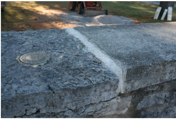
FIGURE 143. A small metal USGS medallion is embedded in the limestone perimeter wall near what used to be the pedestrian entrance for visitors arriving by rail. Source: Stones River National Battlefield, photo by park staff, 2014.
