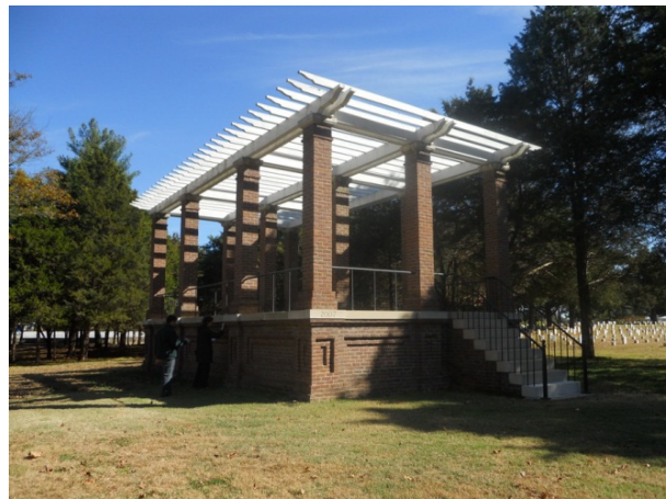
FIGURE 97. The original rostrum was demolished in 1941–1942 due to its poor condition. In 2007, the park reconstructed the rostrum based on original designs for the structure.
