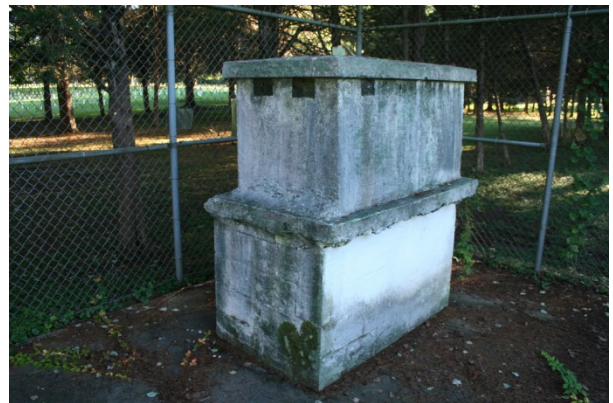
FIGURE 120. The former powder magazine is a concrete masonry structure. Source: Stones River National Battlefield, photo by park staff, 2014.
