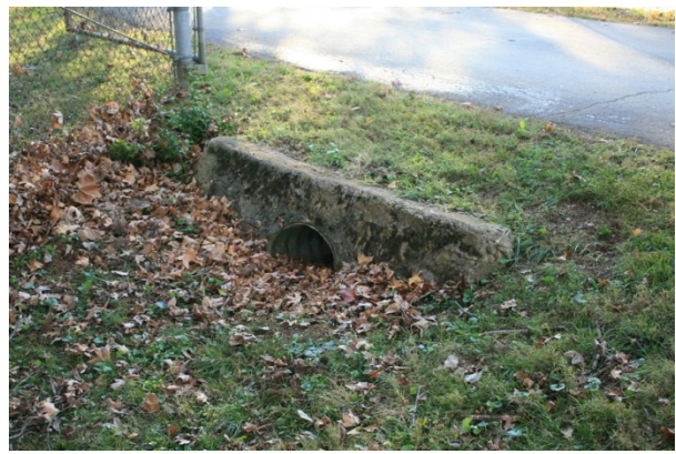
FIGURE 152. A stone-faced headwall and culvert runs beneath the maintenance area access drive just inside the chain-link fence that surrounds the maintenance yard.
