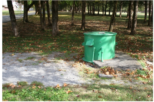
FIGURE 156. A sewer pump station is located beside the gravel access road just inside the maintenance entrance off Old Nashville Highway. Source: Stones River National Battlefield, photo by park staff, 2014.
