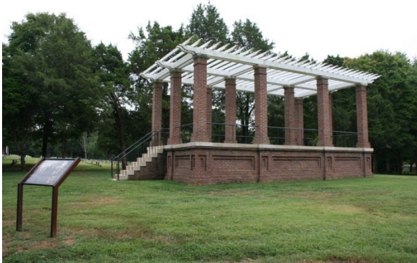
FIGURE 178. The reconstructed rostrum, 2010, view looking southeast. Note the position of the stairs on the eastern half of the north end.
