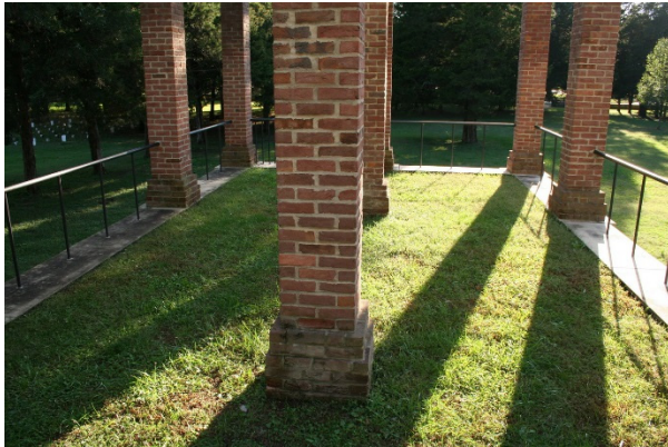
FIGURE 99. Moisture-related staining at the base of the brick posts. Source: Stones River National Battlefield, photo by park staff, 2014.
