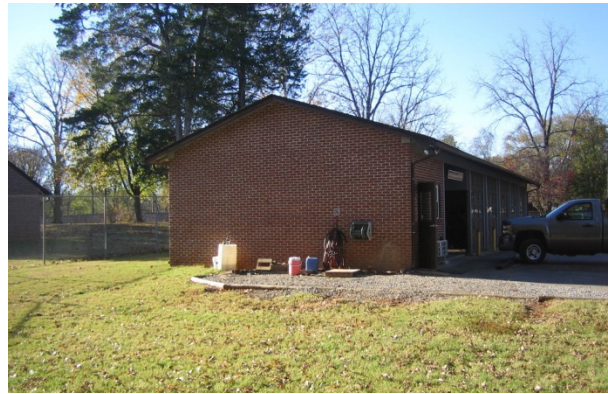
FIGURE 50. The maintenance building before renovation, view from the northeast, November 2010.
