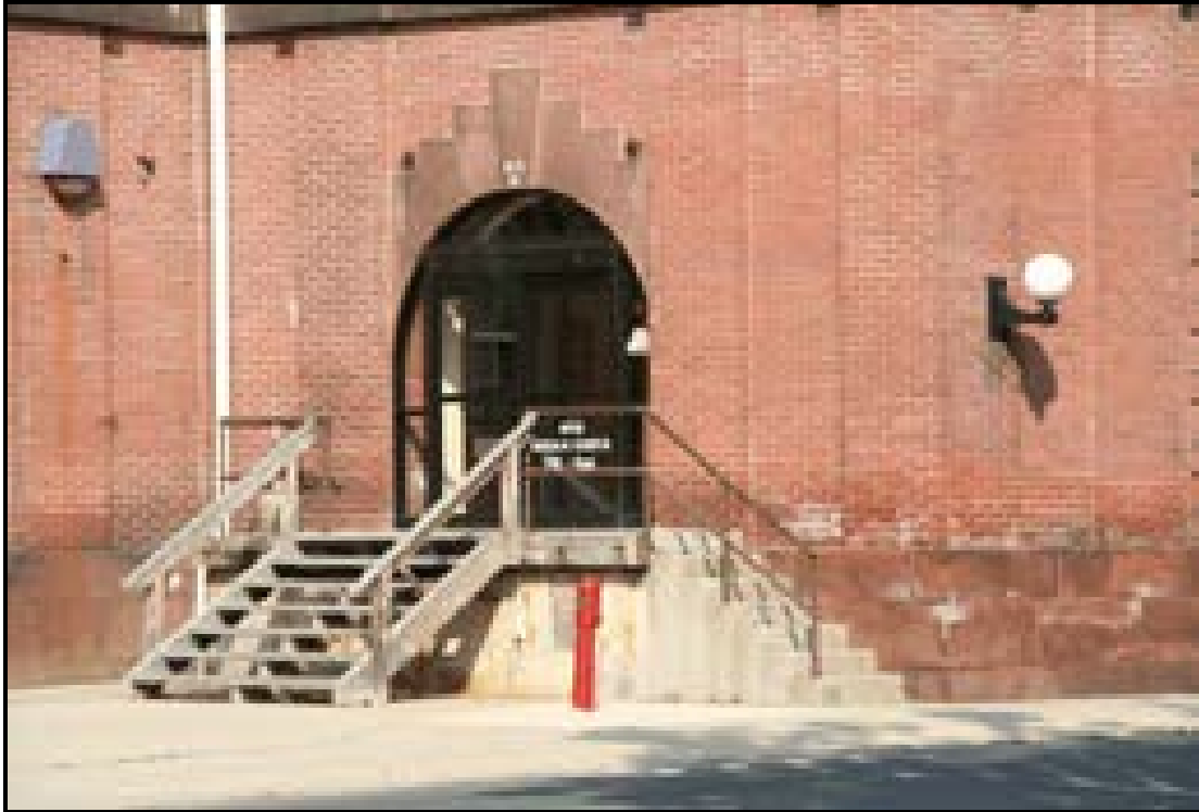
Figure 3.3. Building 13 (Main Arsenal): main entrance with historic concrete loading dock and wooden stairs added for visitors (photo: author).
