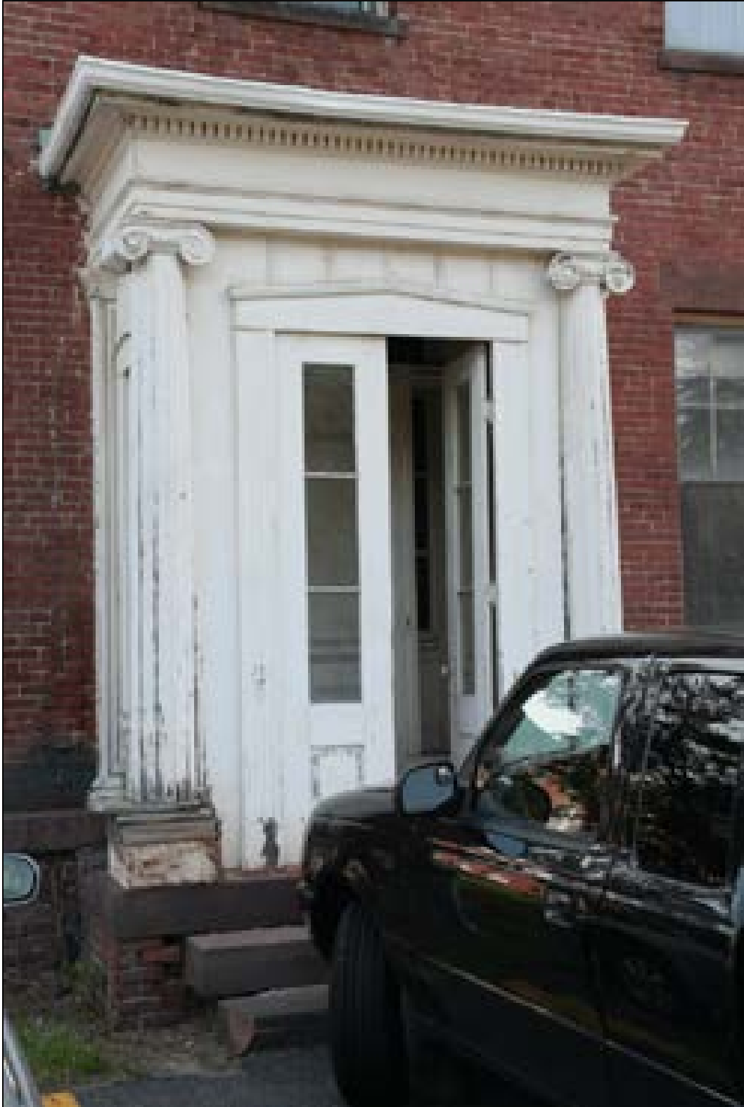
Figure 4.18. The elegant Grecian woodwork of Building 10 is rotting, a missing column base has been replaced by a stack of wooden boards, a sandstone step is overturned. There is nothing to protect the entrance porch from the impact of a carelessly driven car. These conditions, photographed in 2005, had not changed in 2009 (photo: author).
