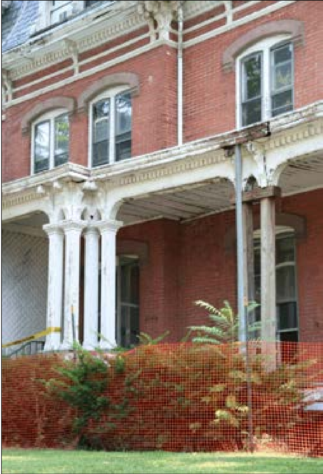
Figure 4.17. Columns are missing from the Victorian verandah of Buildings 5-6. Netting keeps visitors away from the rotten porch floor (photo: author).
