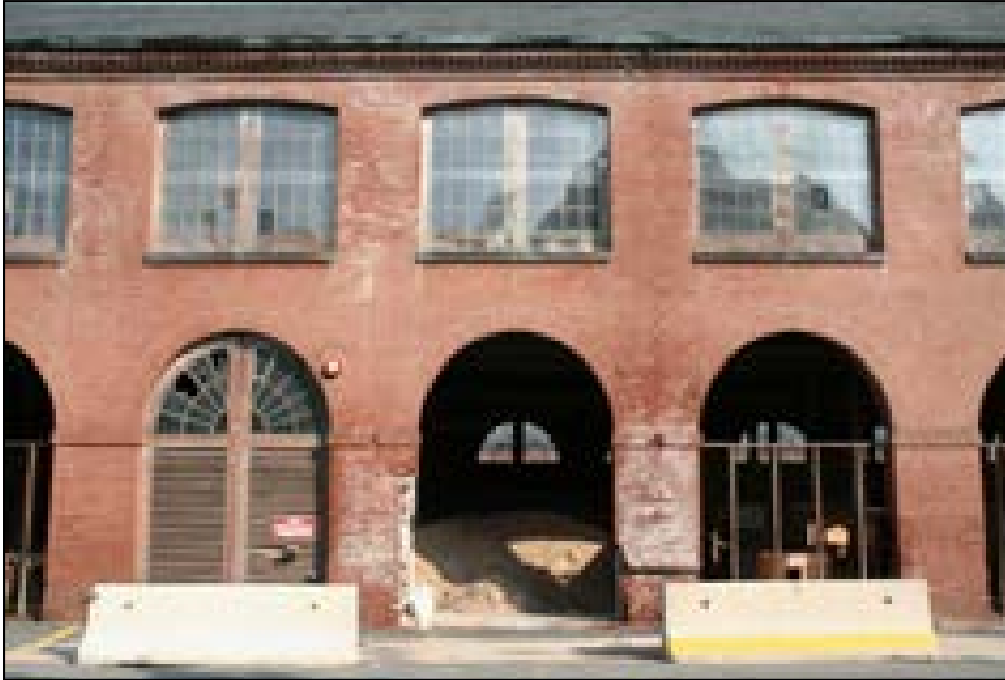
Figure 4.21, In 2005, Building 19 (exterior photo) was open to weather, pigeons and vandals, its interior used for storage of miscellaneous objects. In 2009 the concrete barriers were gone, leaving the brick piers unprotected from cars and trucks (photos: author).
