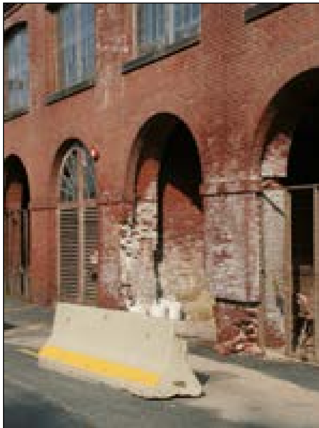
Figure 4.20. At street level, Building 19's brick piers were crumbling (photo: author).
