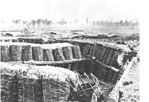
Use of gabions and fascines
