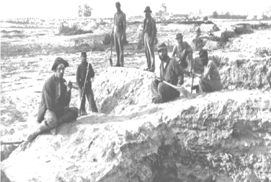
Soldiers constructing earthworks during the war
