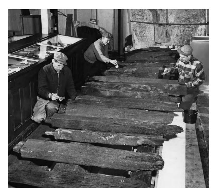
11.3 Workmen applying preservative oil to timbers from the raceway. (Photograph 795a by Richard Merrill, 1953.)
