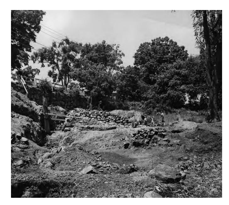
5.1 The excavation of the blast furnace in July 1949. Notice the prominent retaining wall for Central Street at the left of the photograph. The waterwheel and wheel pit were found below the retaining wall. (Photograph 99 by Richard Merrill, 1949.)
