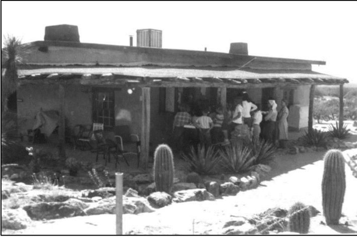
CCC built Administration-residence building and "museum" at Saguaro National Monument. This building was built in the 1930s and has been razed. This "visitor center" was approximately 0.4 miles south of the current VC, and was replaced by the current VC building in 1953. Photofile No. 75SAGU061; SAGU negative no. SAG 297.
