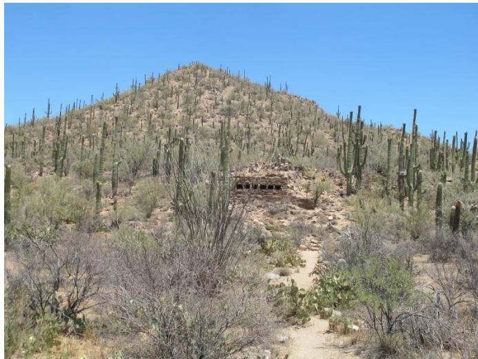
The restroom at Ez-Kim-In-Zin almost disappears in the rocky hillside behind it.
