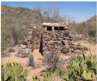
Figure 2. The CCC constructed women's room at Sus picnic area. Note low profile and skirt or stone buttress that ties the structure to the landscape.
