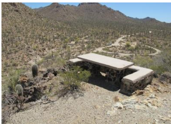
A CCC constructed picnic table with wrap-around bench overlooking Sus picnic area (as seen above) and a view of Avra Valley. The CCC constructed picnic tables were made from local stone with concrete mortar, table and bench tops were constructed of concrete.
