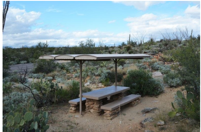
Figure 1. A ramada at the Javalina Picnic Area. The ramada’s roof is constructed from three B-29 bomb bay doors.
