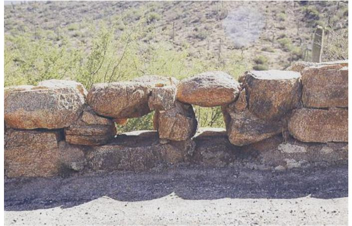
**Close-up of stone capping and water control feature built into retaining wall.**
