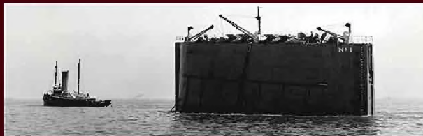
Towing a caisson for the Panama Canal.
