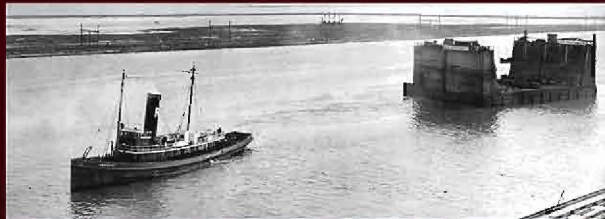
Delivering a drydock section for the Moore Yard, from Seattle to Oakland.
