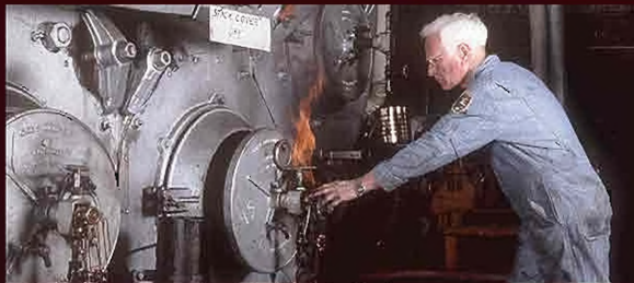
Park volunteer Tom Mac Fadyen lights the oil-fired boiler.
