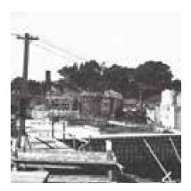
**Figure 18**. By February 1937, crews were framing and completing concrete work for the upper floors of the Bathhouse. (San Francisco Maritime NHP, Historic Documents, Photograph Collection, P88-035.00074)
