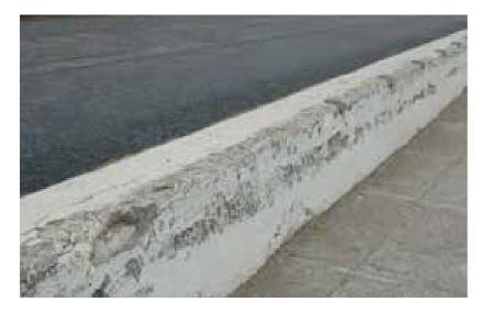
**Figure 96**. Flaking and loss of material along the concrete wall occurs as deterrent bolts fail and water penetrates the under layers of the concrete. Repair may require patching, reapplication of a skimcoat, or some combination. View of the east end of the wall, looking west. (NPS, 2007)
