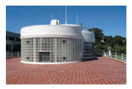
**Figure 55**. Rehabilitation work at the Bathhouse in 2008 included the instillation of a new stainless steel window system; and a modern waterproofing system for the building roofs with new roof tiles to match the historic ones that could not be salvaged. The rehabilitated glass block pantry is now the elevator lobby on the 3rd floor. (NPS, 2008)
