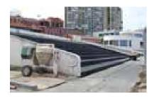
Figure 90. View of the East Bleachers showing new waterproofing material applied during rehabilitation. Note mildew on the concrete wall. Cleaning and repainting this portion of the structure is important to the character of the structure, and should be integrated into overall maintenance. (NPS, 2009)
