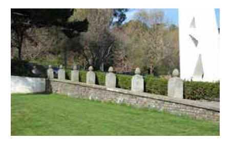
**Figure 98**. View of the stone retaining wall looking northwest from the lawn near the Bocce Ball Courts. The amount of exposed wall visible in the park today generally slopes to the east based on fill added to even the grade when the pump house was removed in the 1940s. (*NPS*, 2008)
