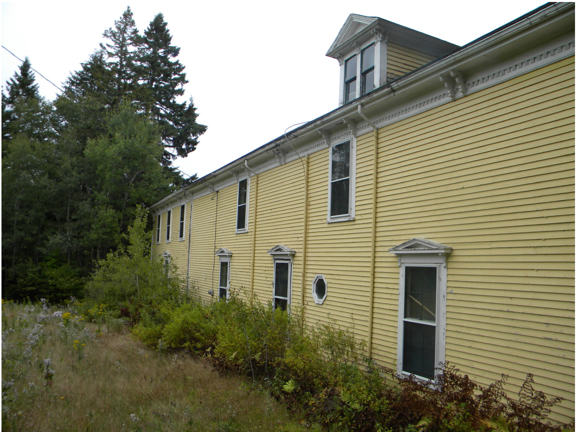
Rear view of the main part of the house
