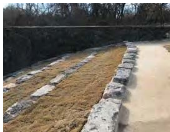
After Landscape and sidewalk rehabilitation at the Espada Aqueduct
