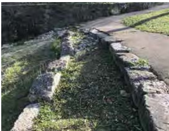
Before Landscape and sidewalk rehabilitation at the Espada Aqueduct
