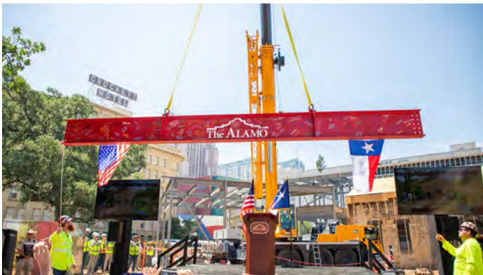
Construction on the Alamo Education Center.
