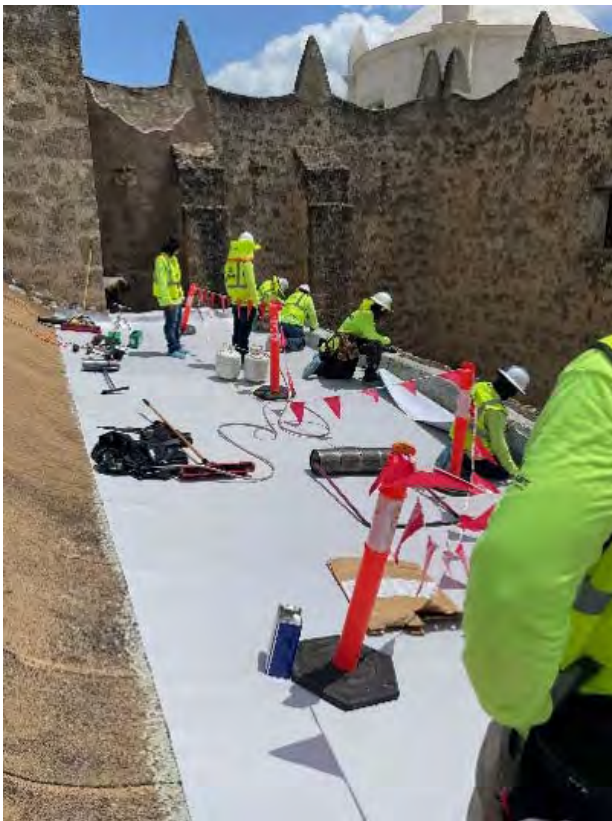
Preservationists work on Mission Concepción's Convento roof.
