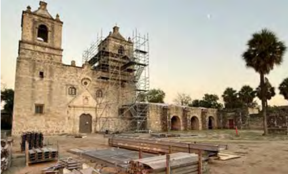
Scaffolding in front of the Mission Concepción Church.
