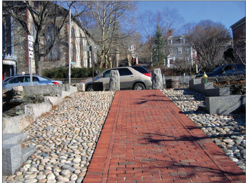
Figure 2.15 (right). The ramped eastern end of Walk F showing its cobblestone shoulders, stone retaining walls, and stone bollards, looking east with St. John's Cathedral in the background, 2008. The treatment of this walk was intended to recall the character of Church Street, which remains across North Main Street. The walk to the Old State House has a similar cobblestone shoulder. (SUNY ESF.)
