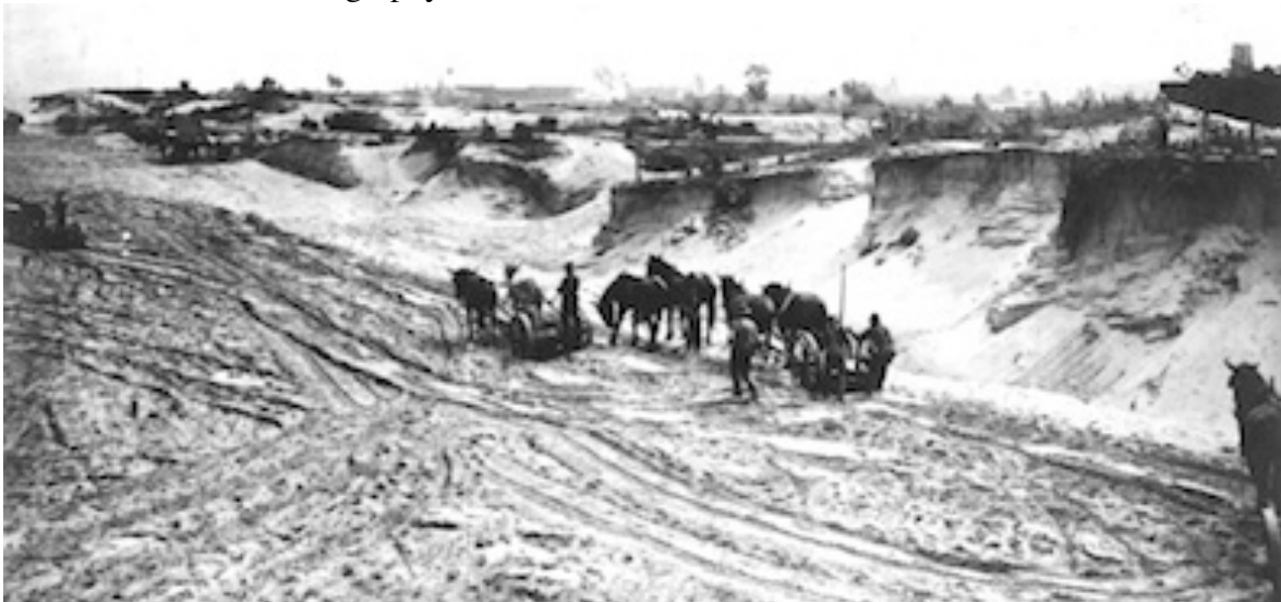
Leveling the dune and swale landscape in 1906 for U.S. Steel's Gary Works.
