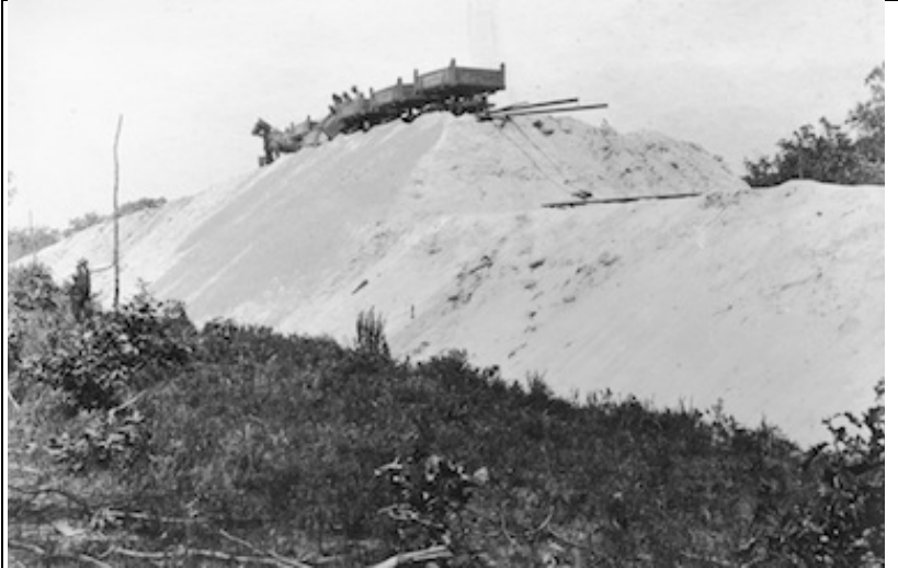
Using dune sand to raise the ground surface for construction of the tracks of the South Shore Railroad, circa 1906. Note that the source of energy is a horse. [Courtesy of Ed Hedstrom]
