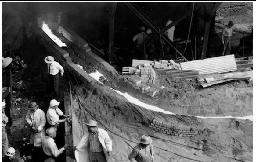
Crisman sand 11 lining the troughs through which molten iron flows from an Inland Steel blast furnace.
