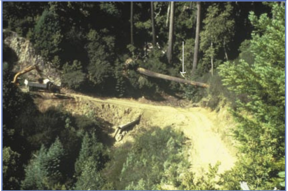
Above: Logging road crossing on Emerald Creek just prior to excavation.
