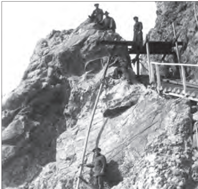
Building the stairs down to the original foghorn building, another 150 feet below the lighthouse level.
