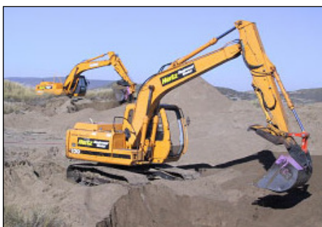
Contract and volunteer crews as well as heavy equipment are restoring dune ecosystems.
