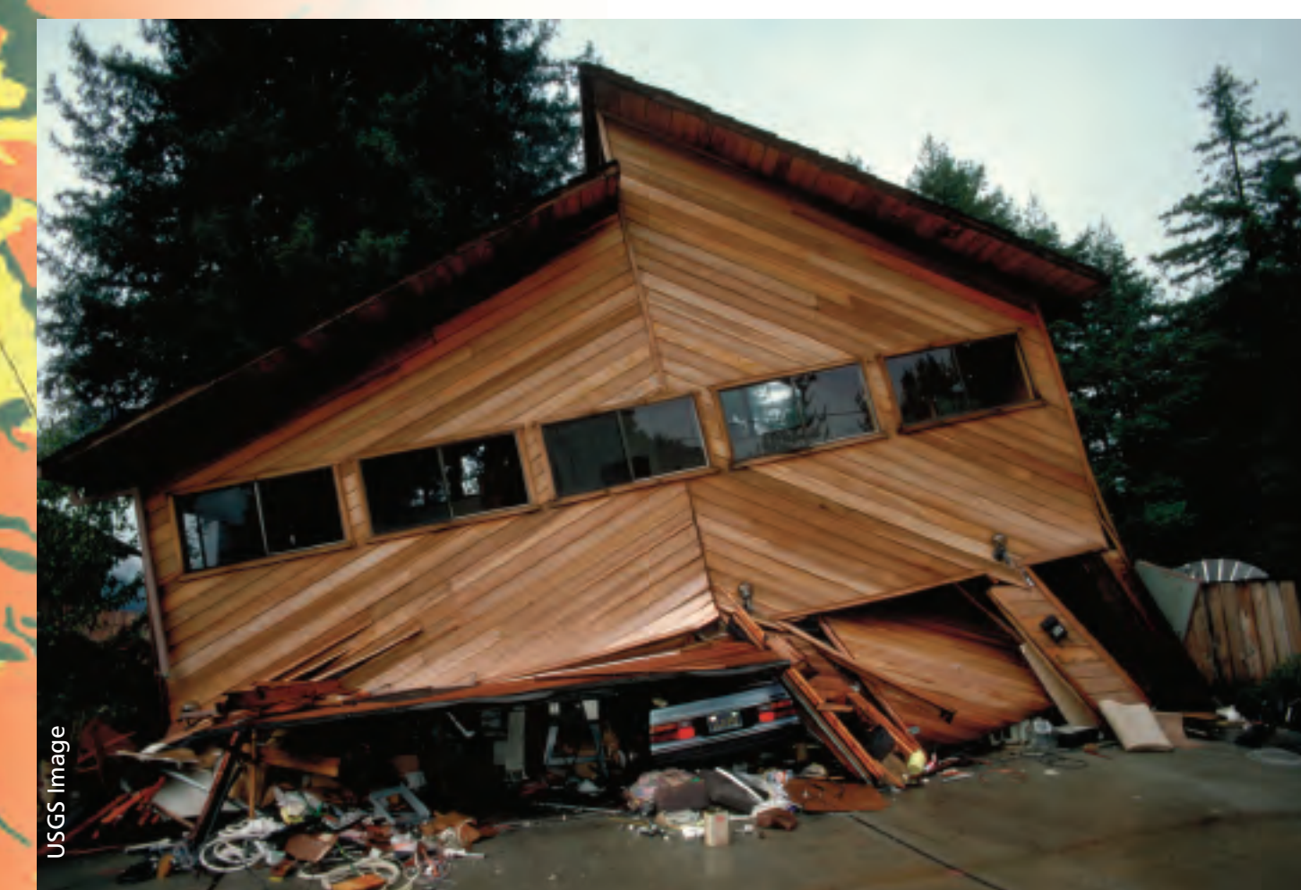
House collapse near Loma Prieta epicenter
