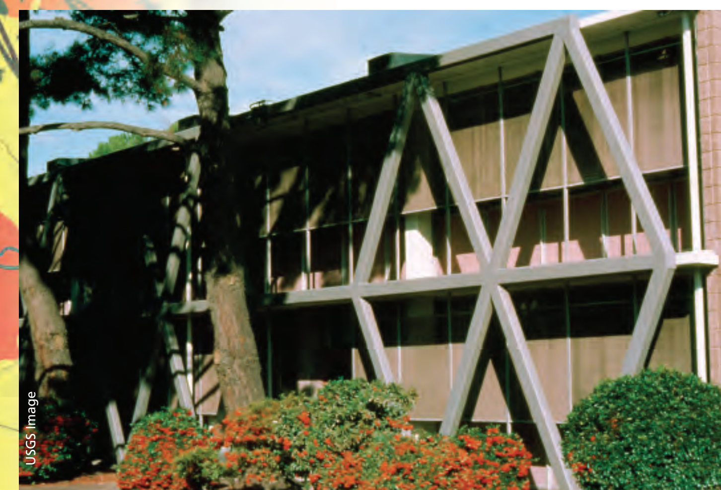
Retrofitting at USGS headquarters
