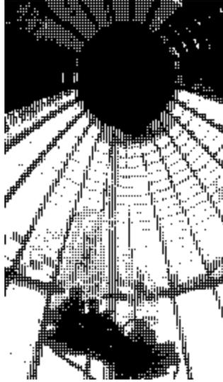
*First-order Fresnel lens seen from inside the lens, Point Reyes Lighthouse. The electric lights are a modern addition.*
