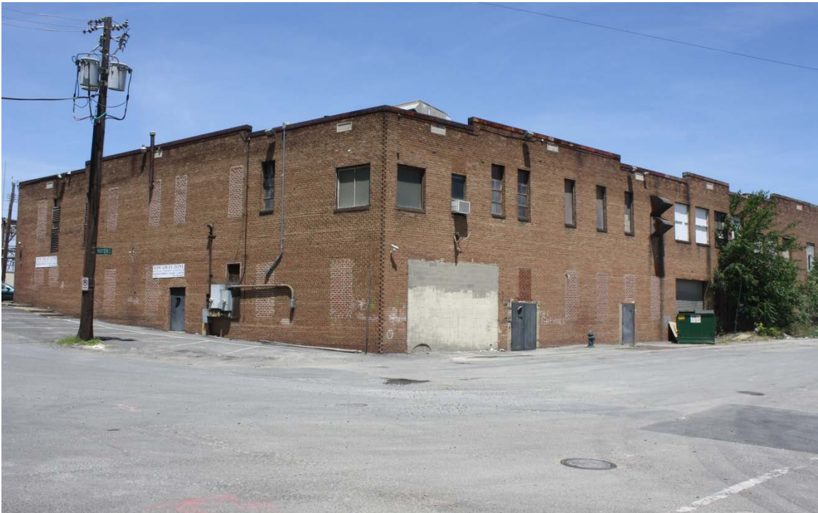
Figure 2: The south and east façades of 1824 Half St, SW (Commercial). Photograph by Lisa P. Davidson, 10 June 2016.
